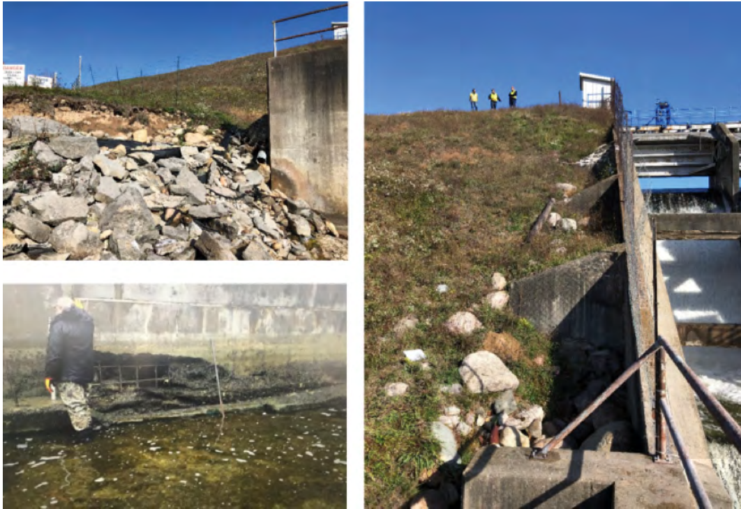
FIGURE 17: Inspection Photographs of Secord Dam
