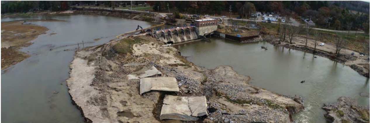
FIGURE 34: Aerial View of Sanford Dam Failure
