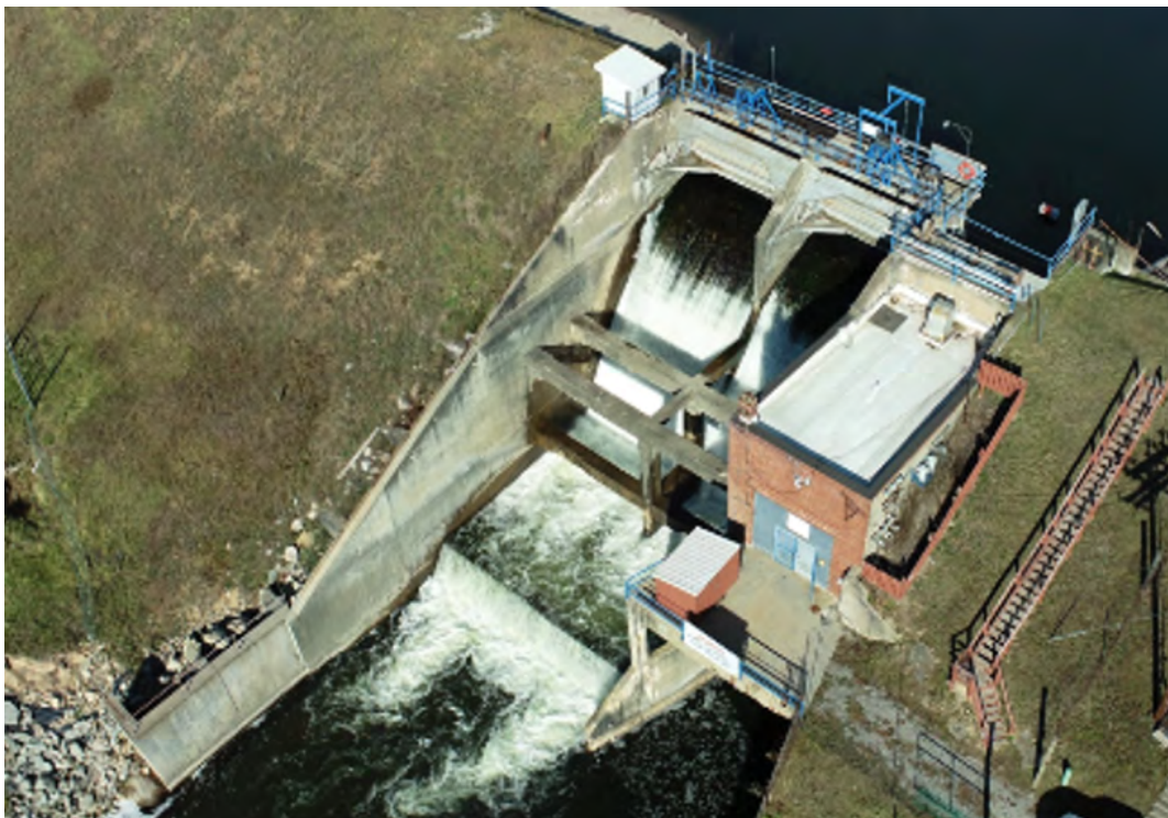
FIGURE 16: Aerial View of Secord Dam Spillway and Non-Operational Powerhouse
