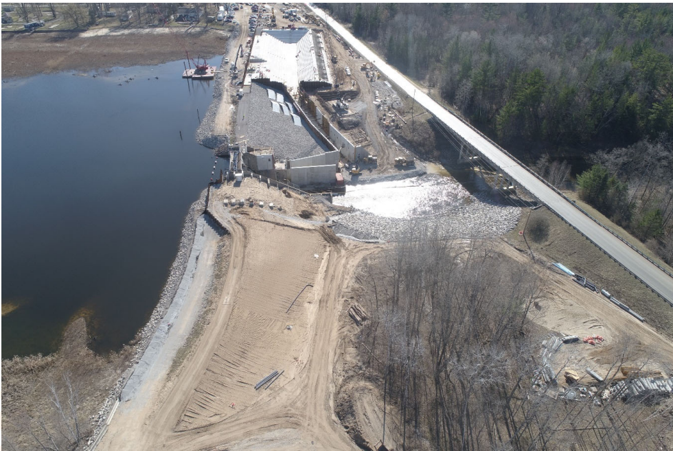
Secord Dam – Looking East
