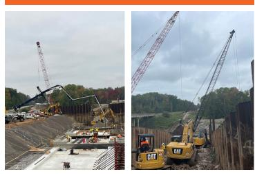
Concrete pours on the stilling basin continue. The lower level outlet demolition and concrete pouring are still ongoing but making good progress. Upcoming is the lower spillway chute that started excavation this week and we will be starting the micropile installations on the right abutment.
