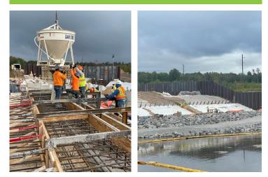
There is a lot of concrete pouring taking place at Smallwood Dam. Areas with ongoing concrete pouring include the lower level outlet walls, upper chute stilling basin, baffle blocks, and end still (pictured left). Pictured right is a crew pouring concrete for the lower spillway chute.
