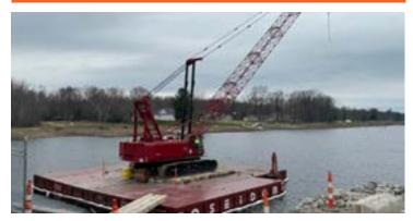
Secord concrete work is nearing completion in the stilling basin and the auxiliary spillway chute. We are installing soil anchors in the auxiliary spillway now. Low level outlet concrete work is ongoing. Upstream, we have the crane and barge (pictured above) mobilized for cofferdam installation and dredging work to begin. The right embankment work is ongoing as we install tension anchors for micro-pile installation.
