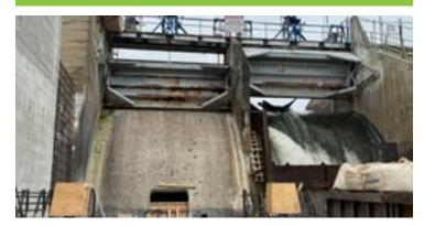
The work on Smallwood is progressing very well with completion of phase 1 and 2 on the cofferdam. Our team successfully diverted water using the siphon system to dewater the area around the dam to start concrete work. Demolition work on the existing powerhouse is still ongoing. The flood door for the auxiliary spillway is being installed. We are still working on the downstream right abutment grading and slope work.
