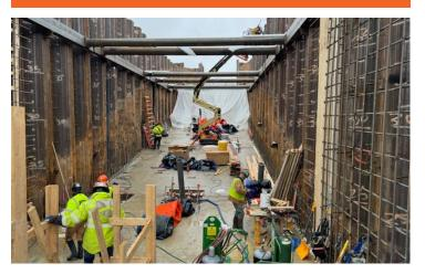
We are continuing to to prepare, form, and pour concrete in the auxiliary spillway chute. Prioritizing snow removal is an added step before continuing to pour concrete. Excavation is ongoing in the auxiliary chute area. Crews are also continuing demolition and restructuring in the low-level outlet. Armoring the west embankment is nearing completion. Work will continue as long as the weather allows.
