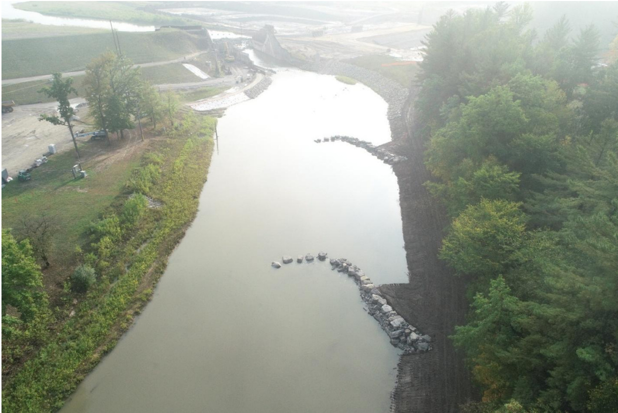
Figure 5: J-hooks in downstream Edenville Dam improve riverbank instability and erosion.
