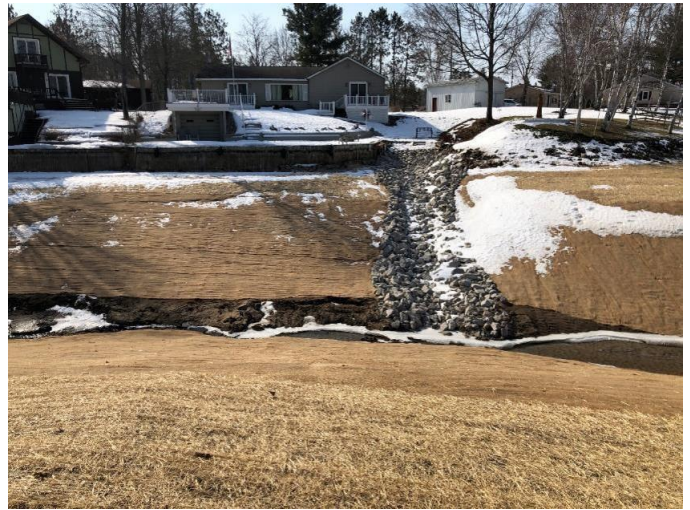
Before and after erosion mitigation on Anderson Drive as part of the Natural Resources Conservation Service Emergency Watershed Protection program conducted after the flood.
