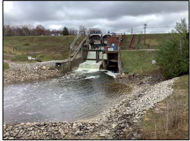
Photo 6.1-4. Secord Dam, facing north.
