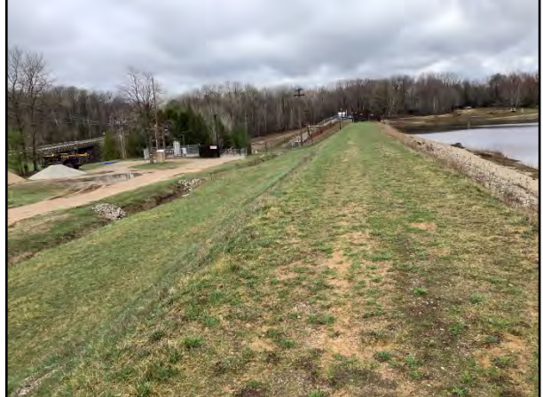
Photo 6.1-2. Eastern berm flanking Secord Dam, facing west.
