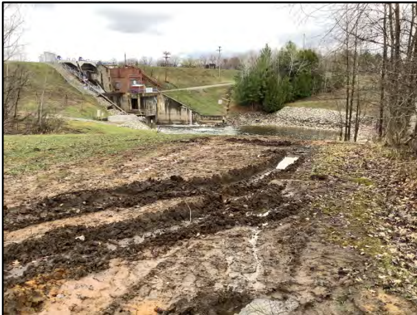
Photo 6.1-5. Recent access road disturbance, facing east.
