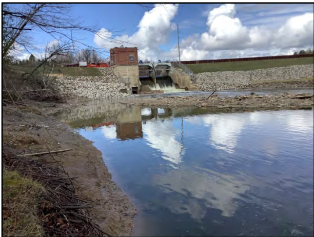
Photo 6.2-3. Smallwood Dam, facing west.
