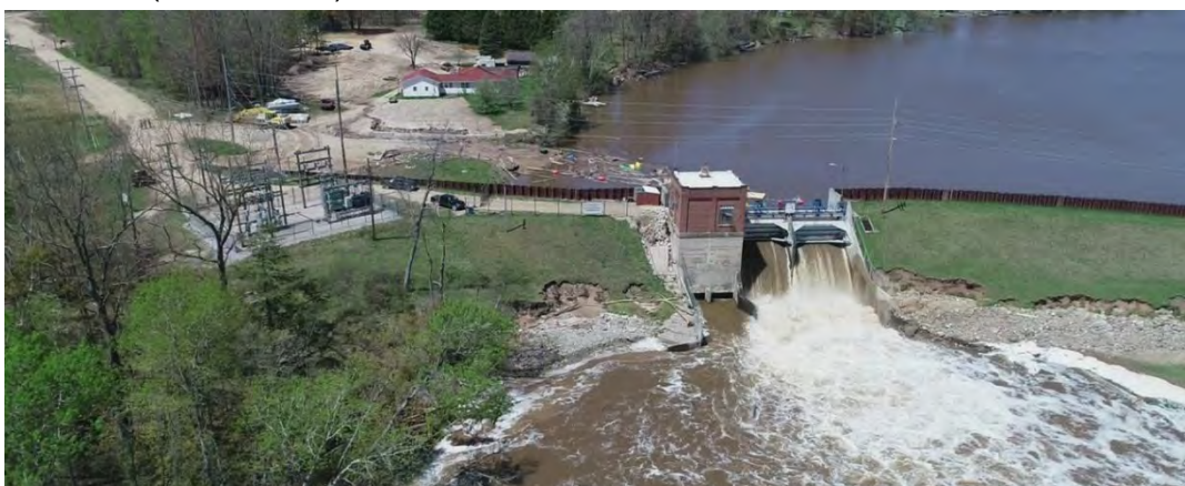
Photo 3. Aerial Drone Imagery of Smallwood Dam, May 2020.
