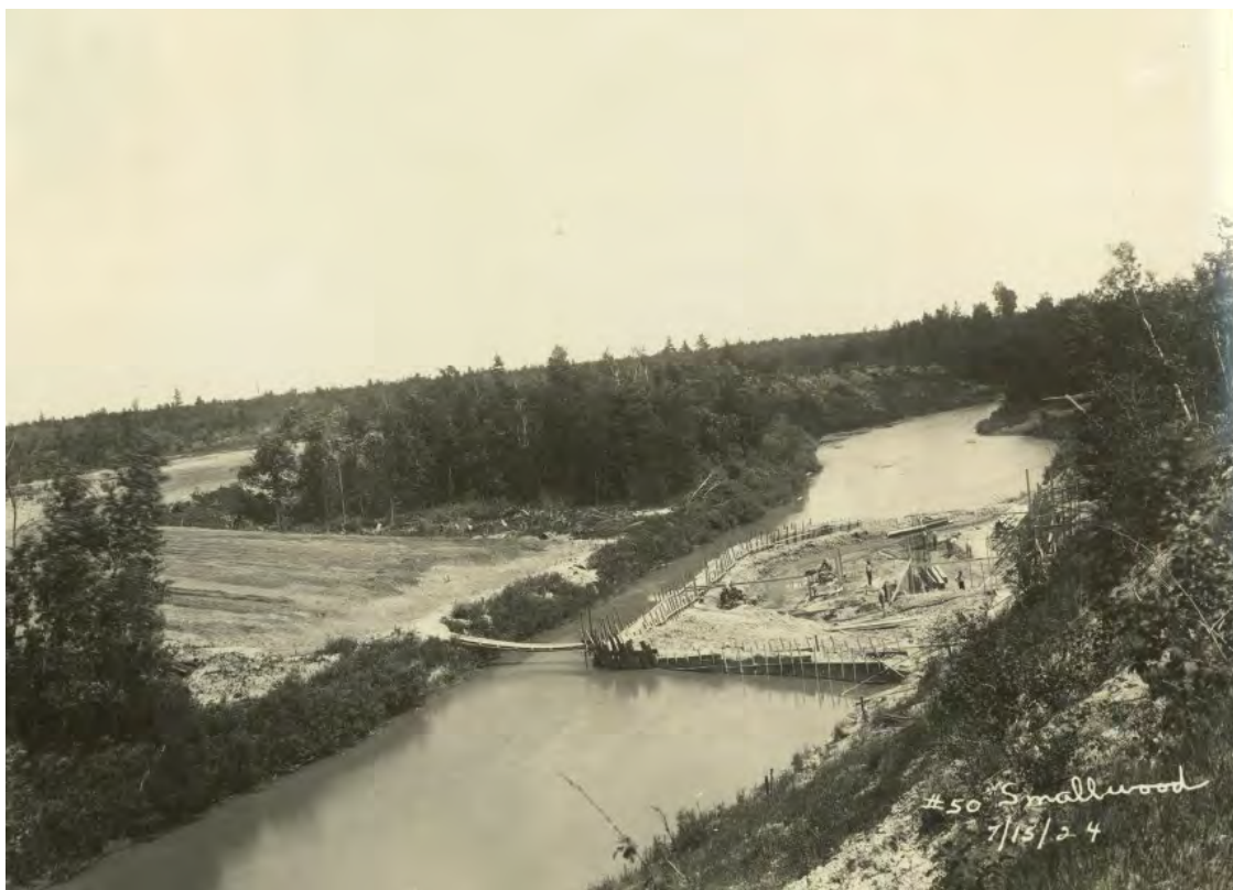
Photo 4. Smallwood Dam During Construction, 1924.
