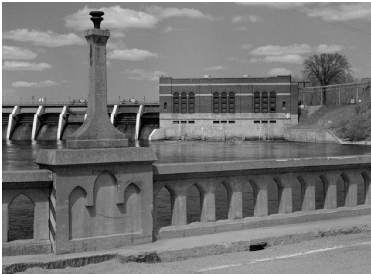
Photo 6. Chalk Hill spillway (left) and powerhouse (right).
