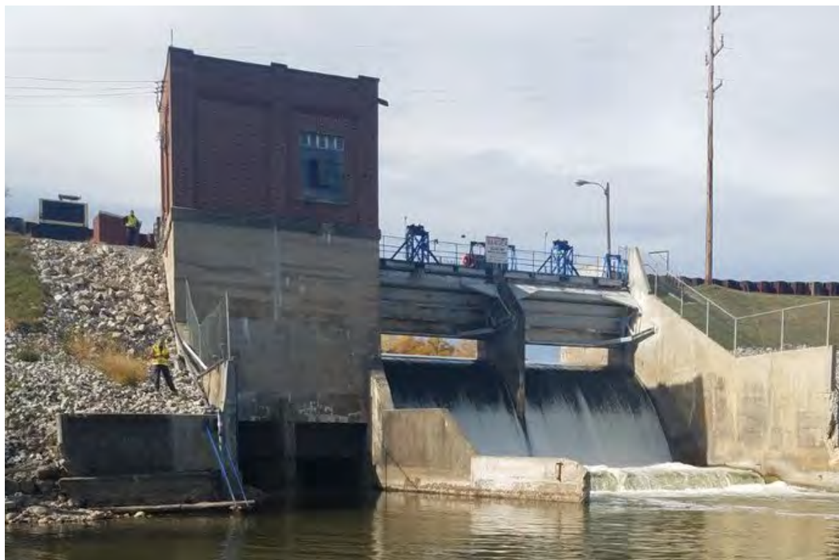
Photo 1. Smallwood Spillway and Powerhouse, October 2020.
