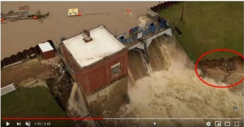
Photo 7.6: Overtopping of spillway left training wall during May 2020 event.
