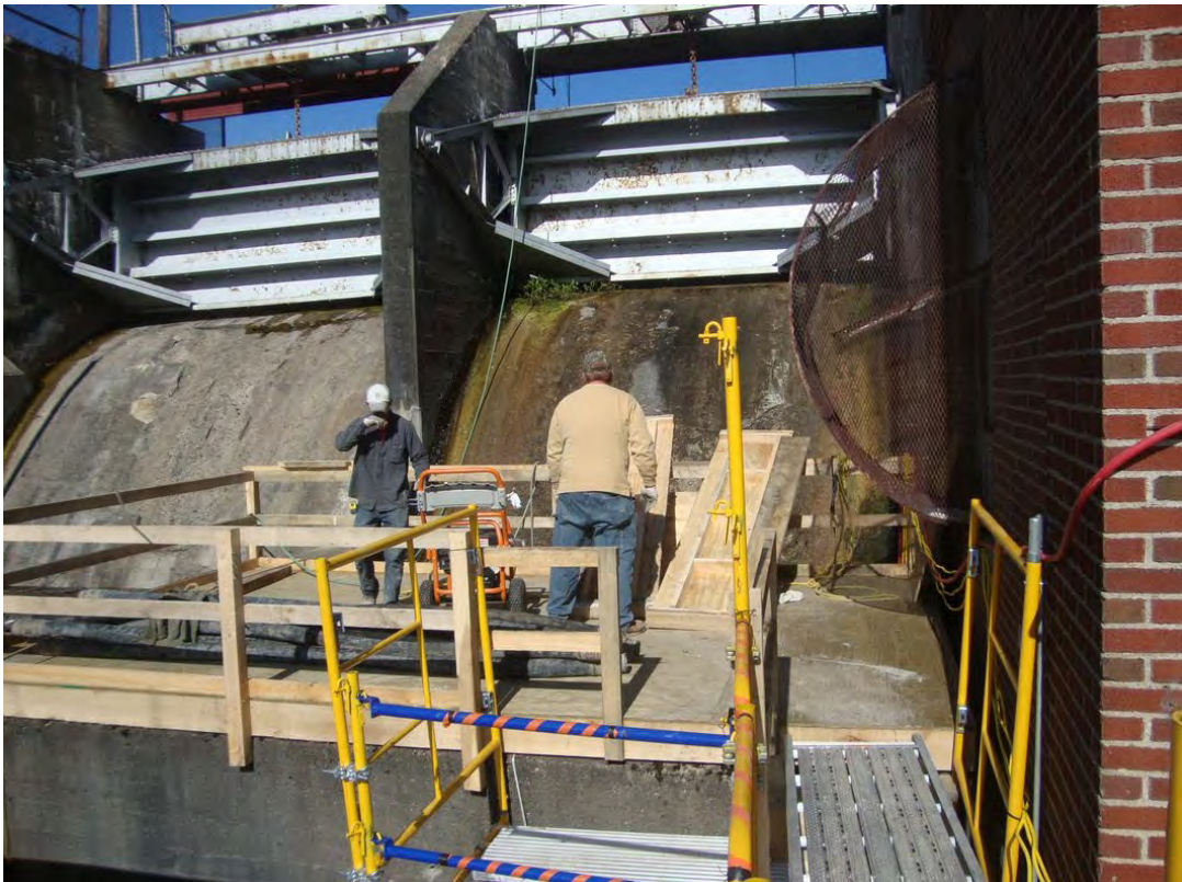
Photo 8. Spillway Resurfacing, 2012.
