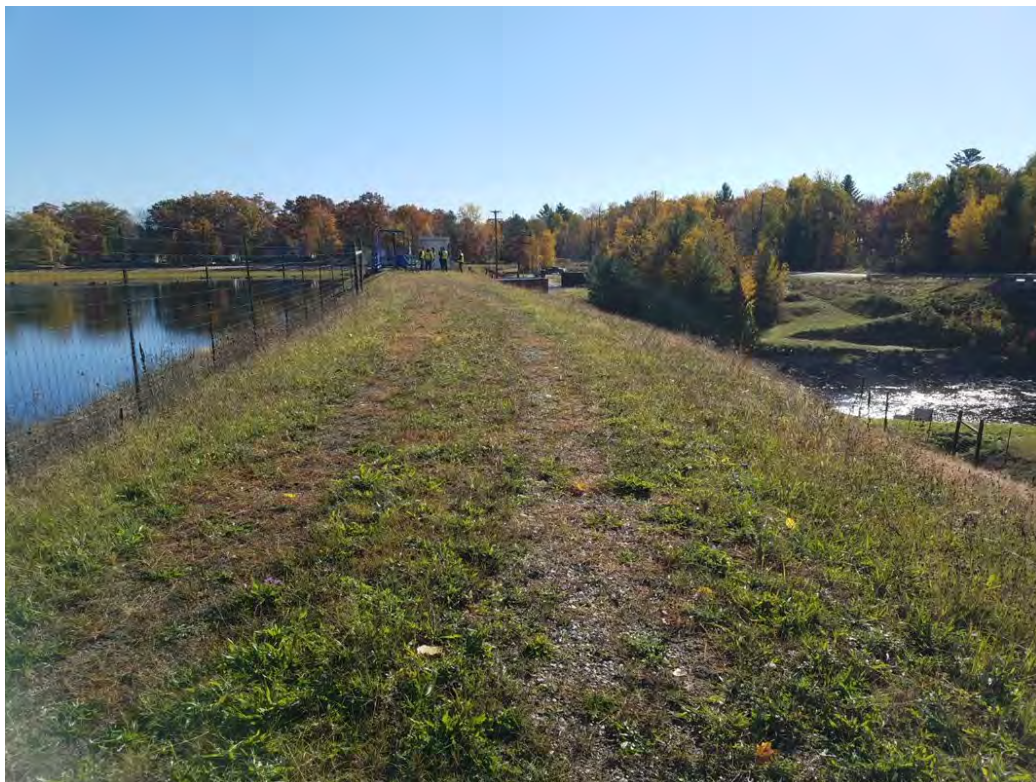
Photo 4. Secord Dam Left Embankment, 2021.
