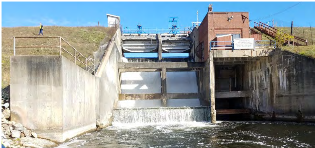
Photo 1. Secord Dam Overview, May 2021.
