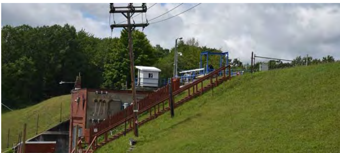
Photo 3, Secord Powerhouse and Left Embankment, August 2019.
