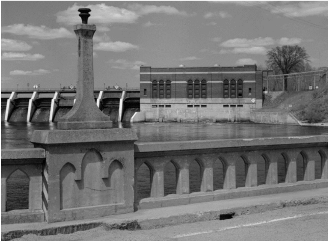
Photo 9. Chalk Hill spillway (left) and powerhouse (right).
