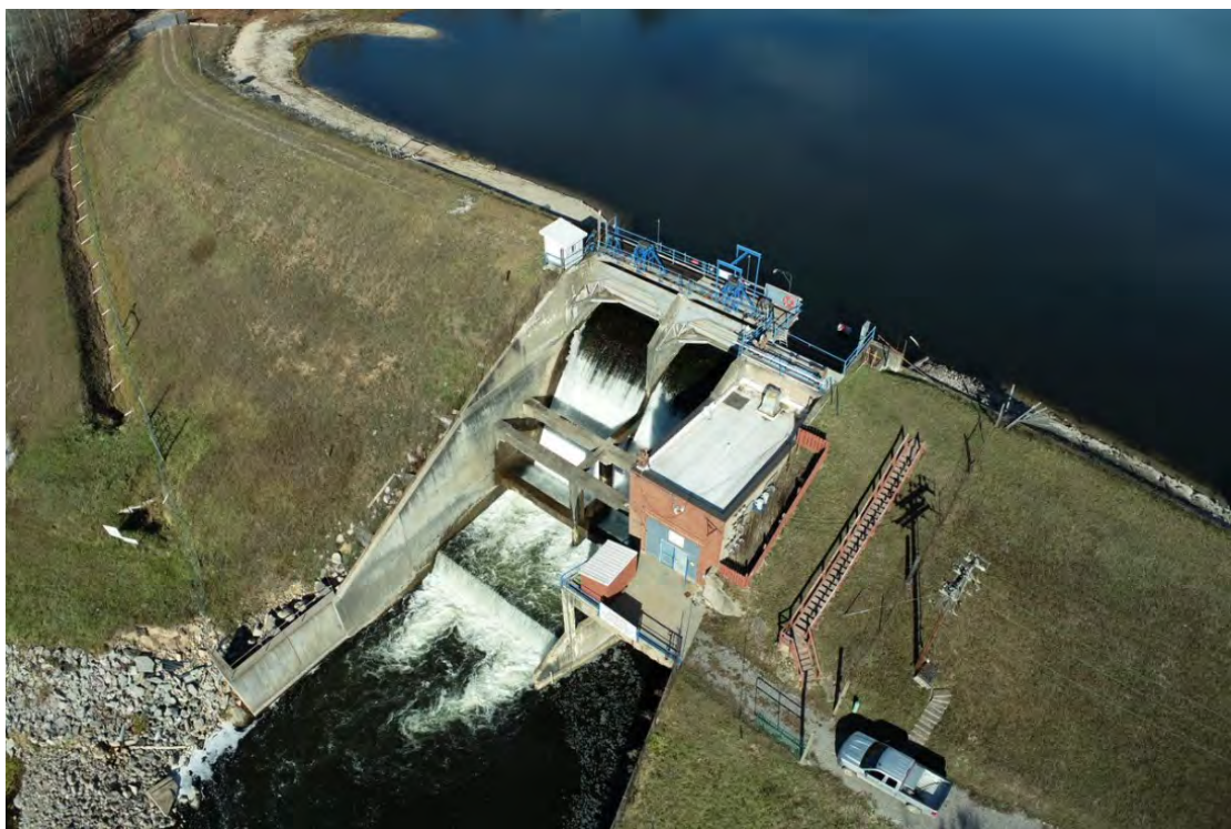
Photo 5. Aerial Drone Imagery of Secord Dam, 2020.
