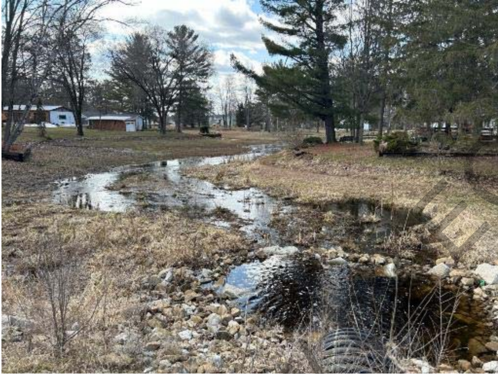
Site 12 – Looking downstream from Poplar Dr.
