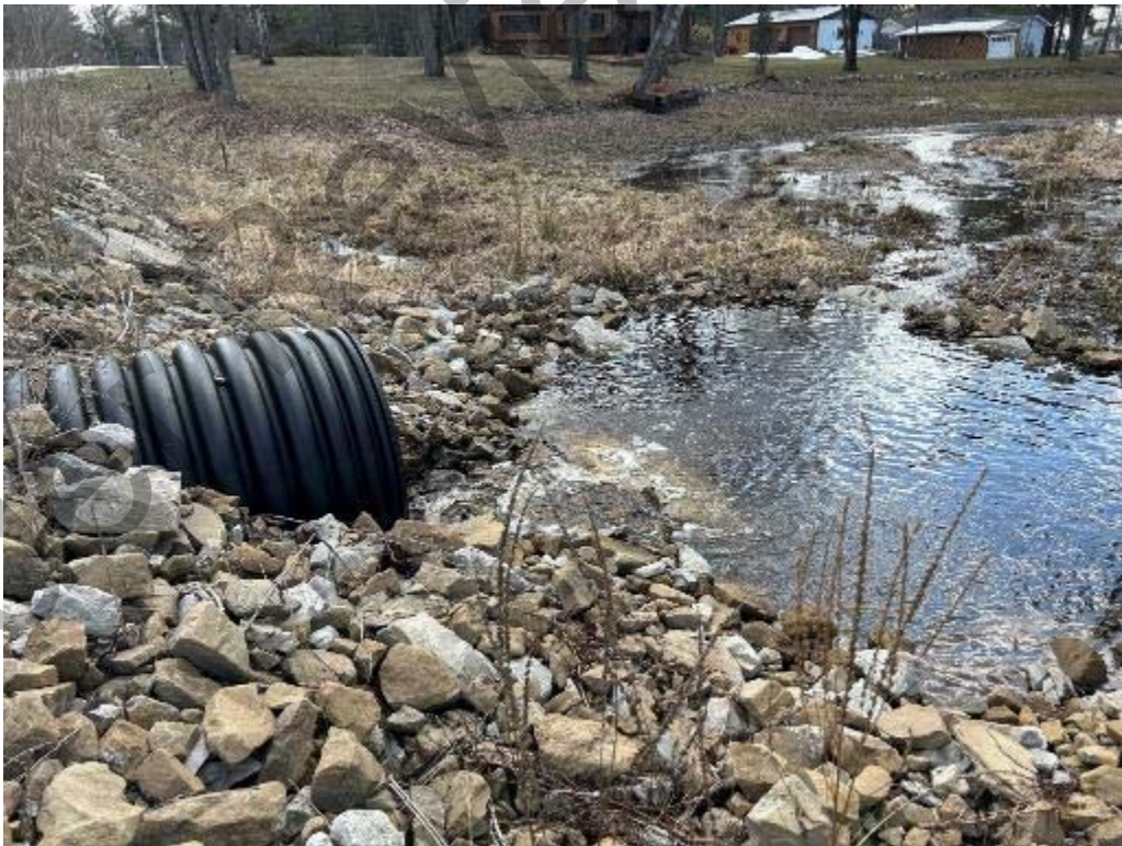
Site 12 – Downstream end of culvert beneath Poplar Dr.
