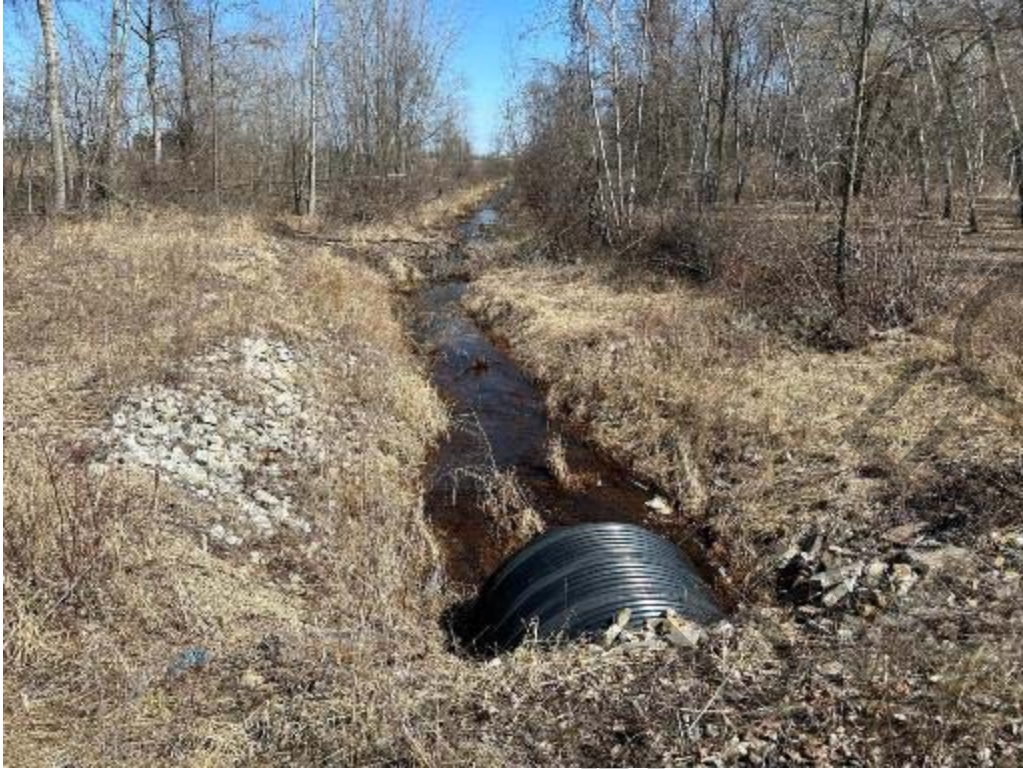
Site 8 – Looking upstream from Red Oak St.
