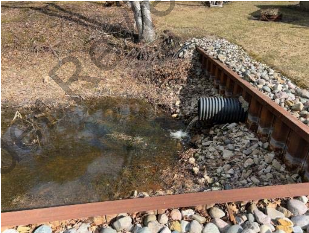
Site 16 – Southern culvert on E. Lakeshore Dr.
