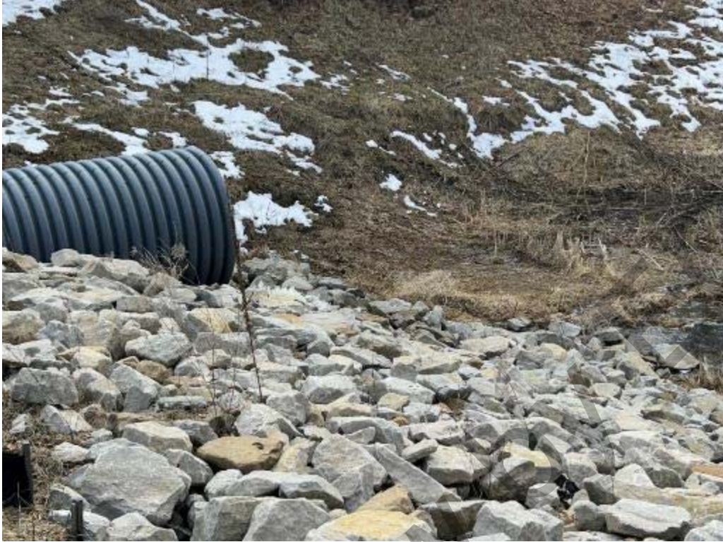
Site 16 – Culvert on downstream side of E. Lakeshore Dr.
