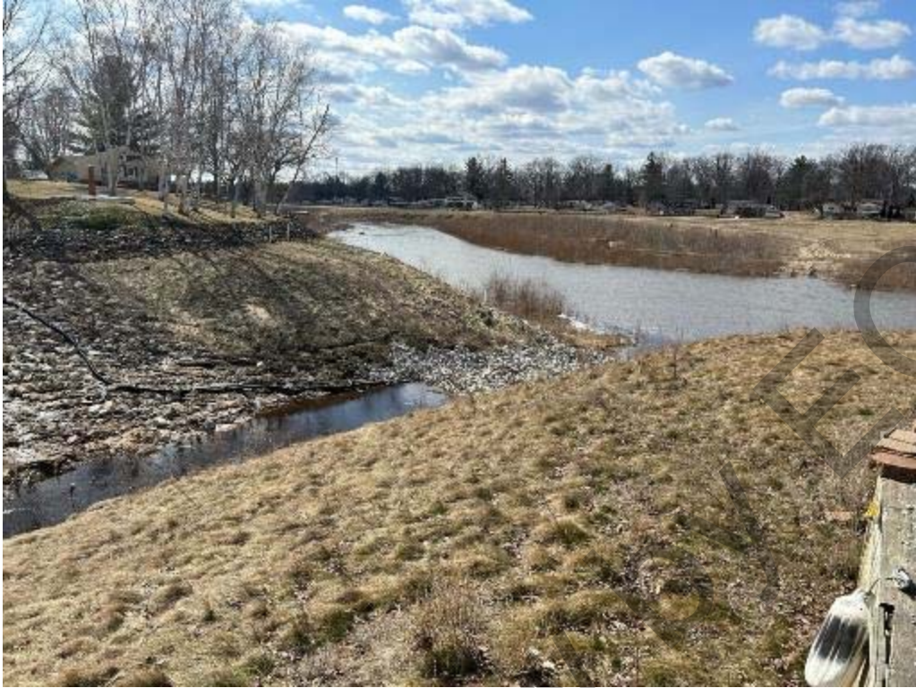
Site 10 – Looking downstream at rock grade control and Tittabawassee River.
