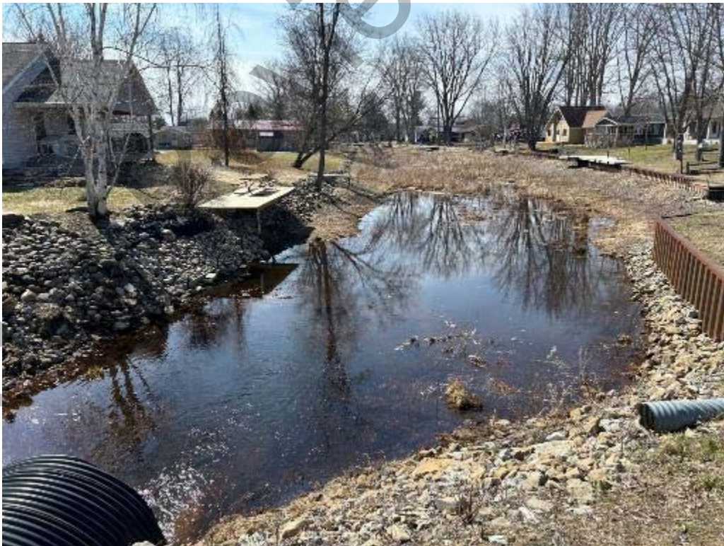
Site 8 – Looking downstream from Red Oak St.
