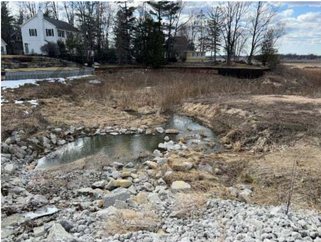
Site 17 – Looking downstream from N. Meridian Rd.
