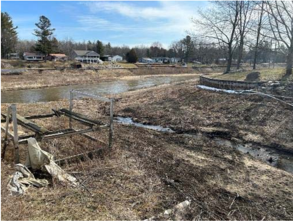
Site 2 – Looking downstream.
