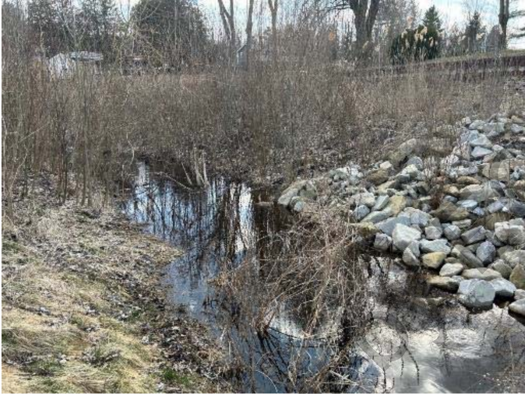
Site 14 – Looking upstream from grade control.
