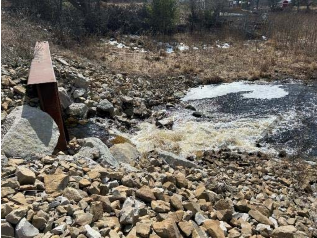
Site 9 – Crossing under Denton Creek Rd.
