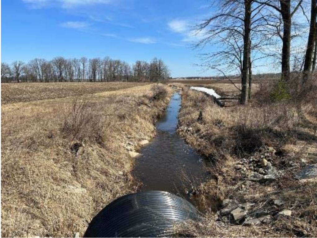
Site 7 – Looking upstream from Red Oak St.
