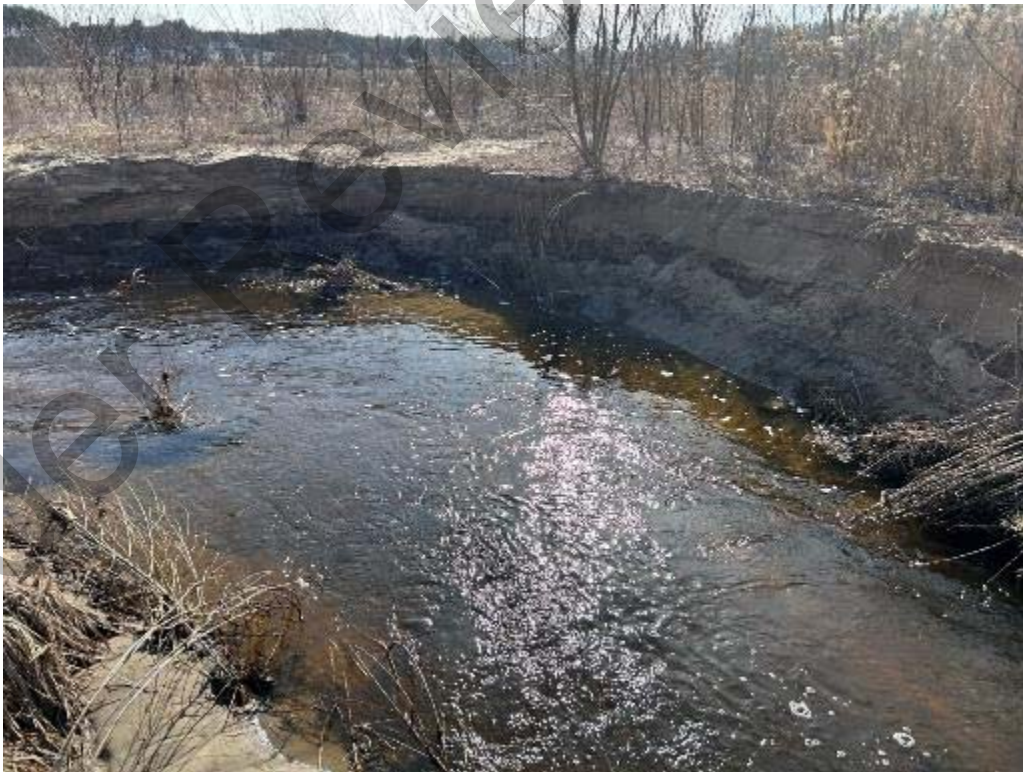
Site 1 – Severe bank erosion.
