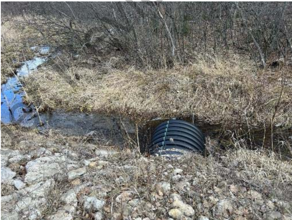
Site 12 – Upstream end of culvert under Poplar Dr.
