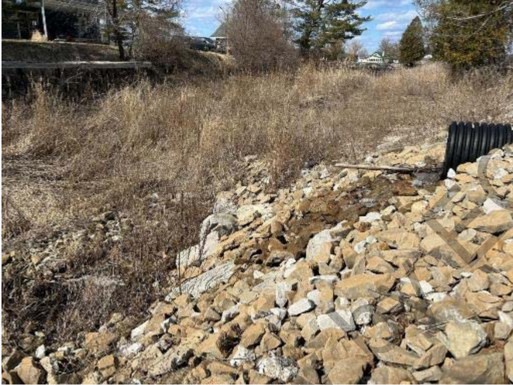
Site 13 – Downstream end of culvert beneath Middle Rd.
