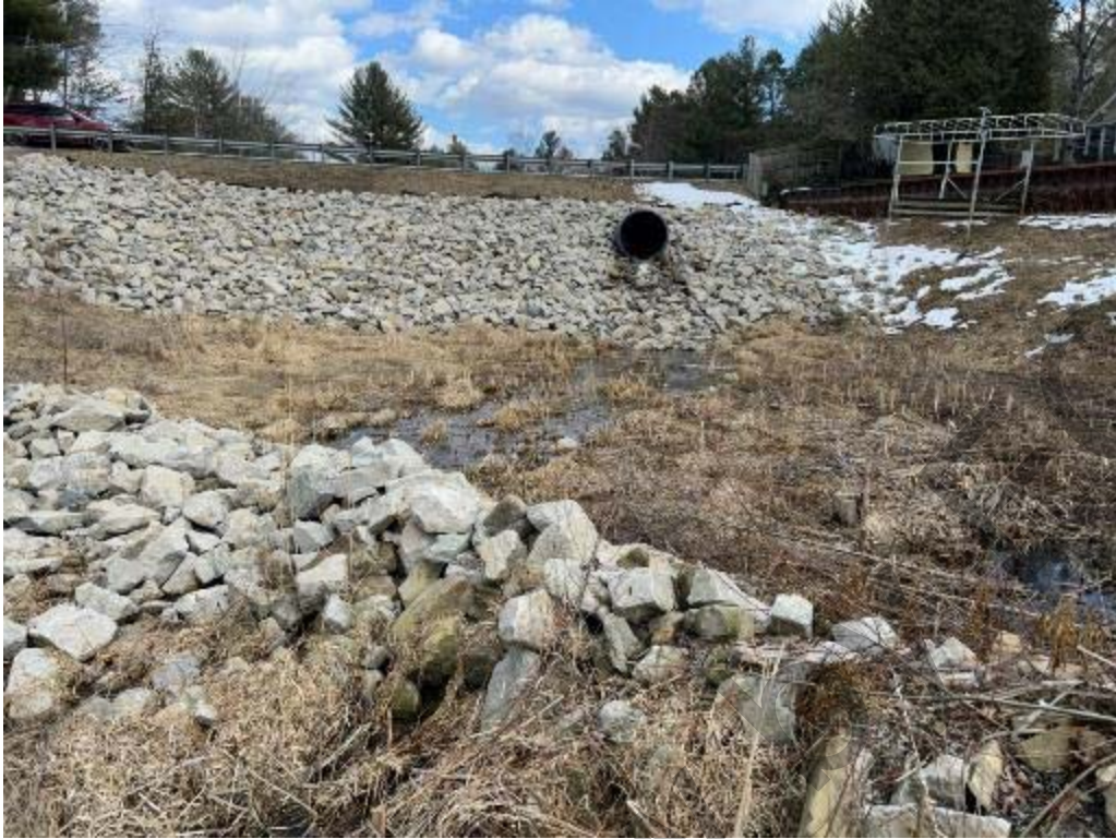
Site 16 – View upstream toward culvert under E. Lakeshore Dr.
