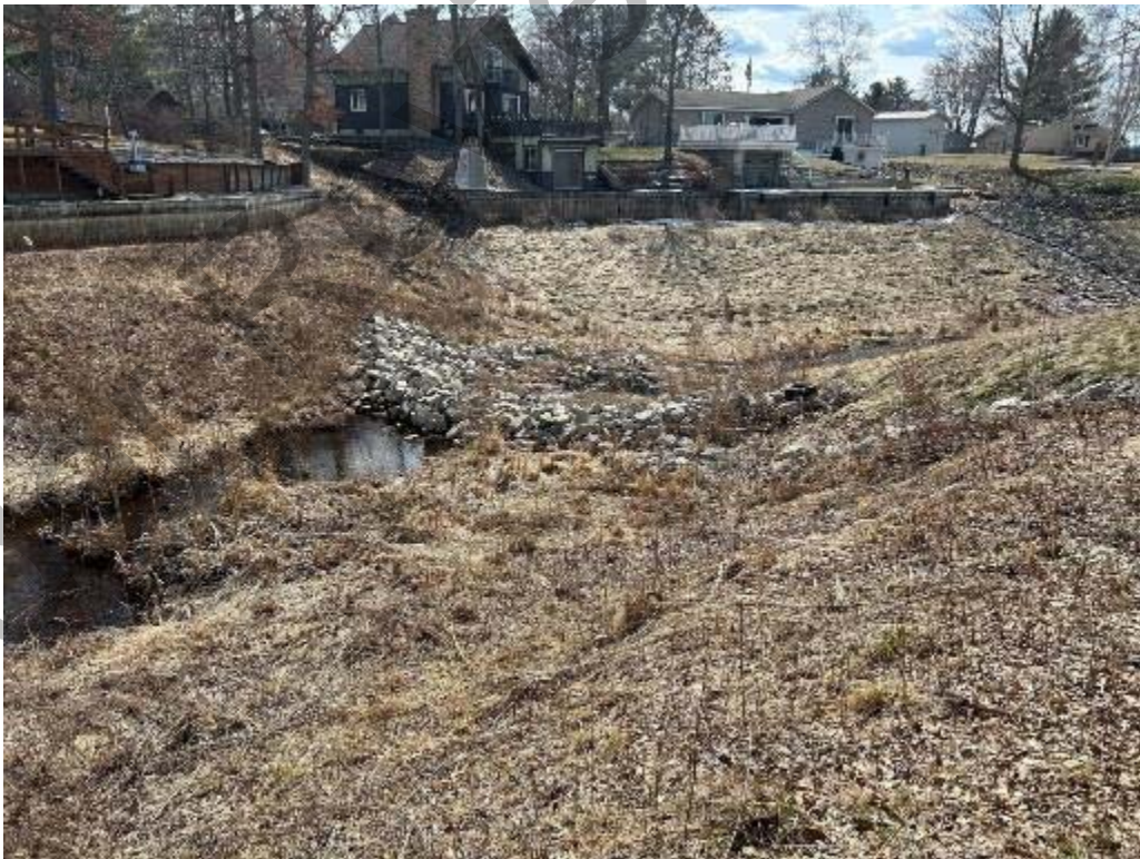
Site 10 – Looking downstream at rock grade control.
