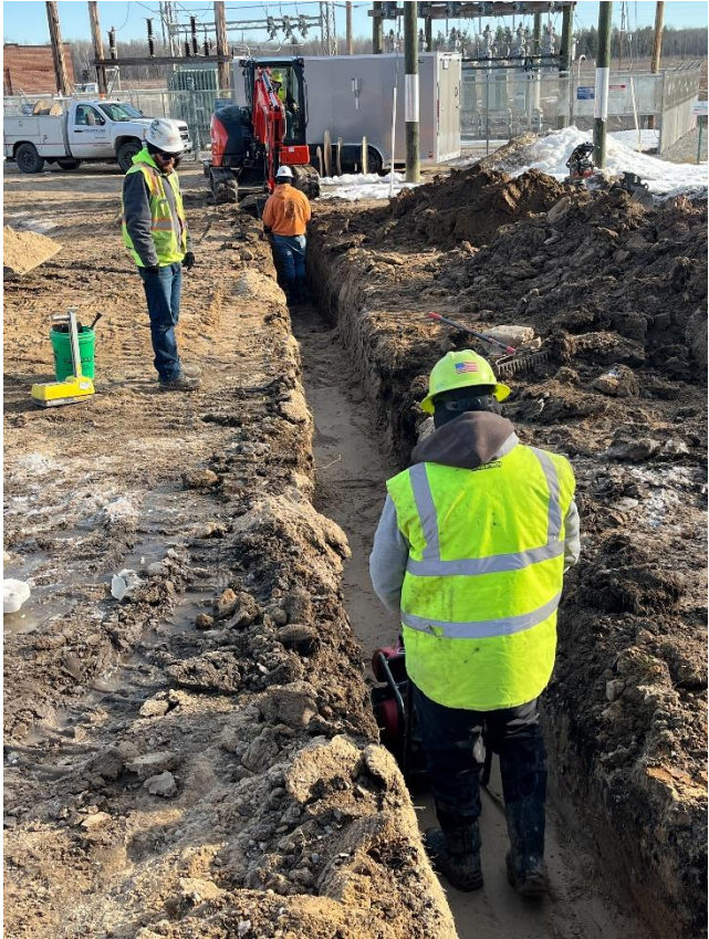
Compacting sand at the bottom of a trench – Smallwood Dam site
