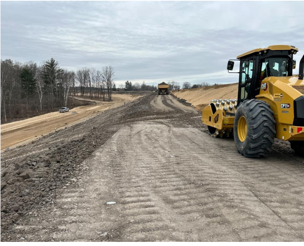
Phase IV – Embankment Restoration – Looking West
