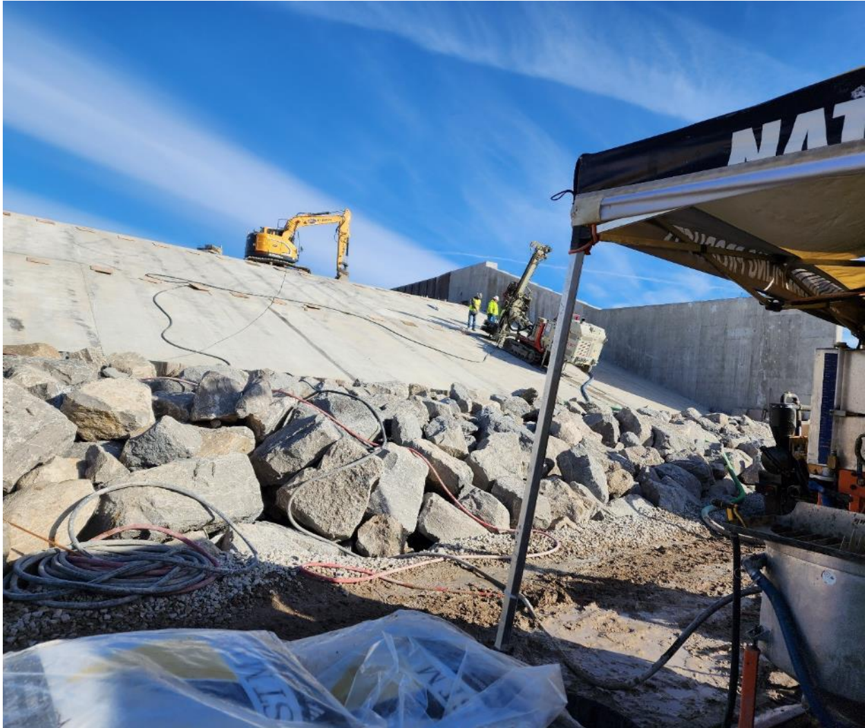
Auxiliary Spillway – Lower Chute, looking North
