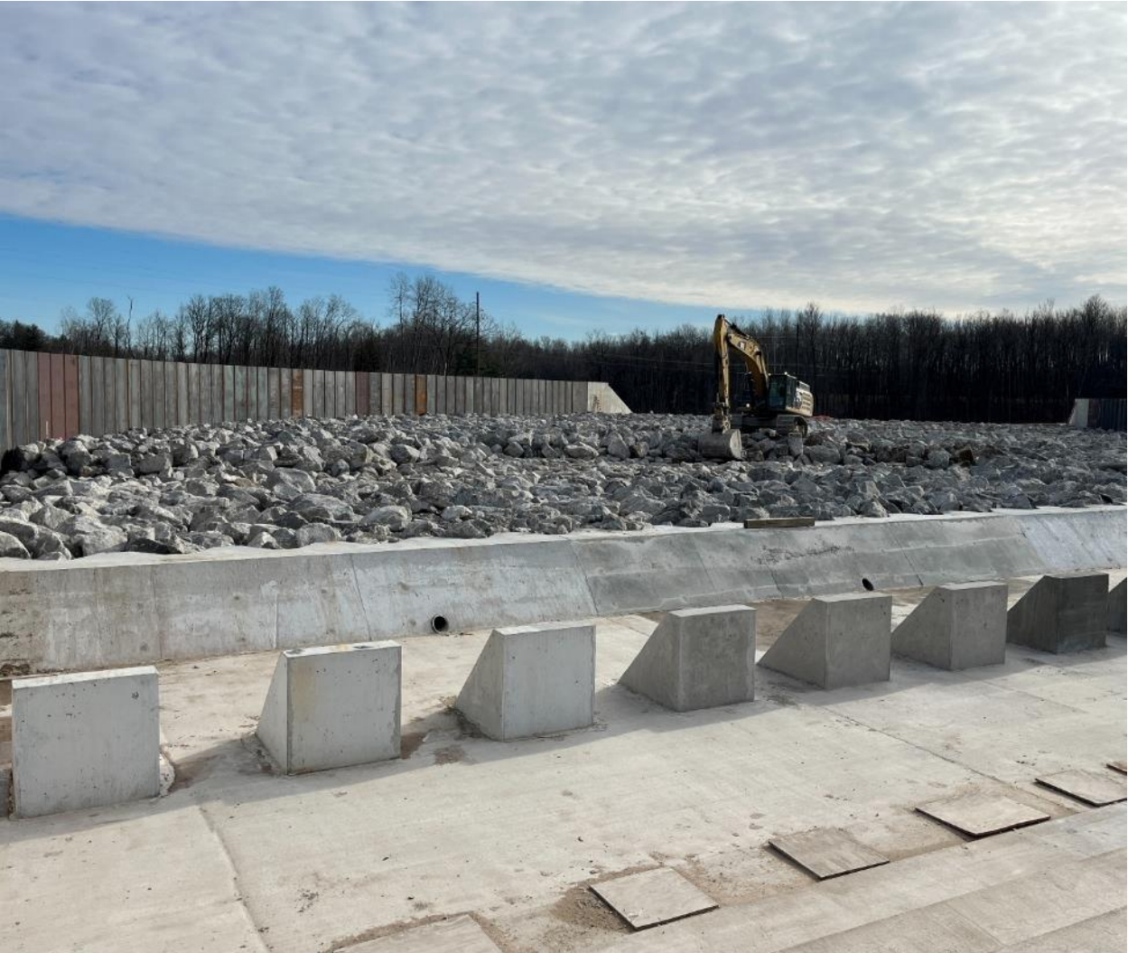
Auxiliary Spillway – Looking East
