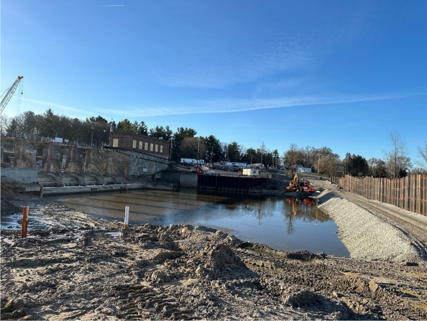
Downstream Cofferdam Area – Looking South
