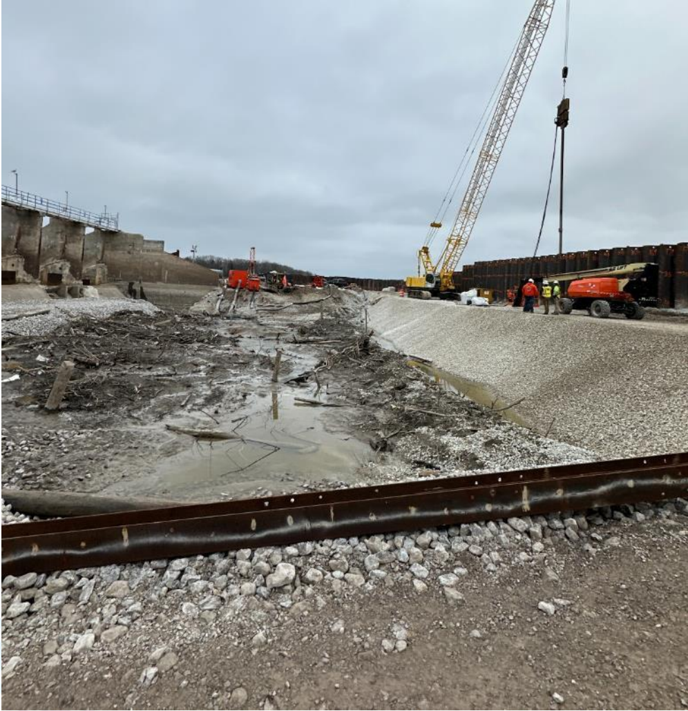
Upstream Cofferdam Area – Looking North
