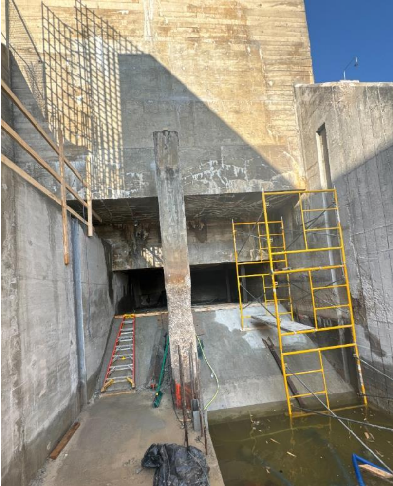
Low Level Outlet Area – Looking West
