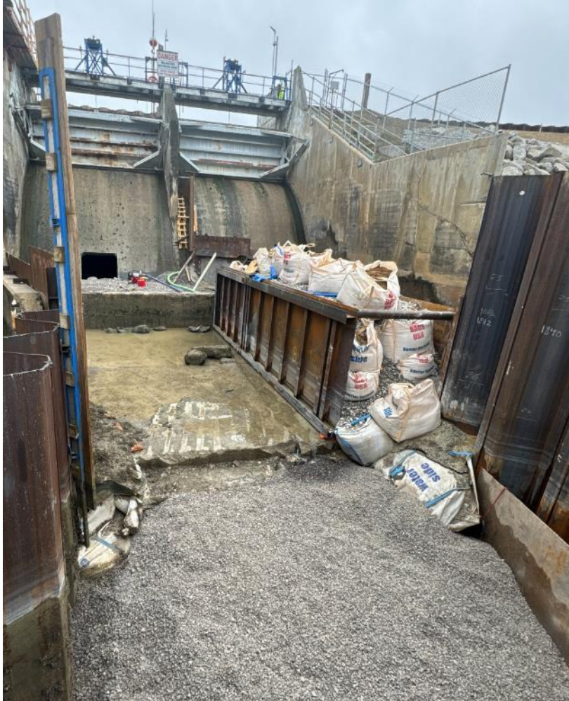
Downstream Cofferdam – Looking West
