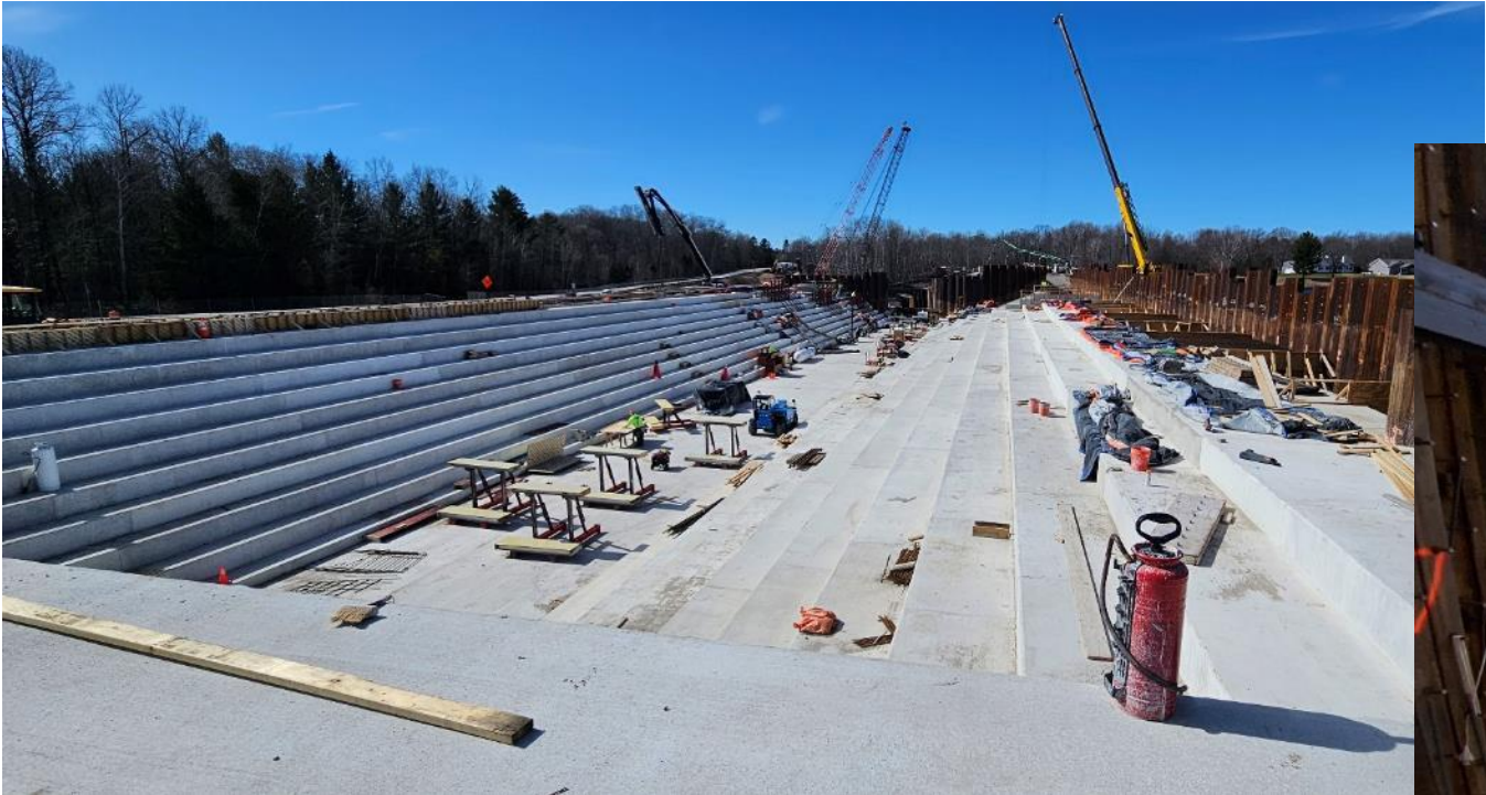
Auxiliary Spillway Basin – Looking west
