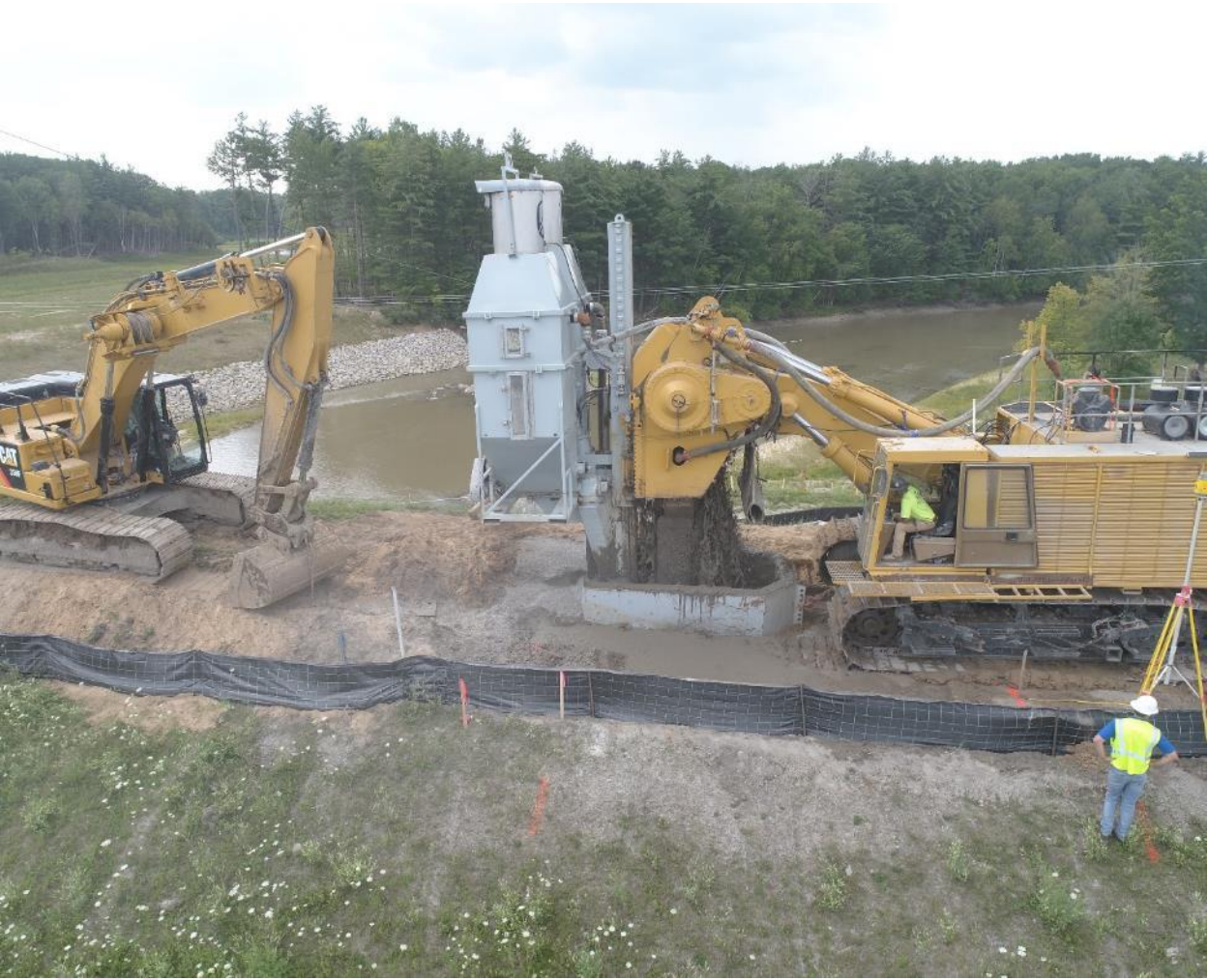
Soil-Cement-Bentonite Wall Installation – Looking South
