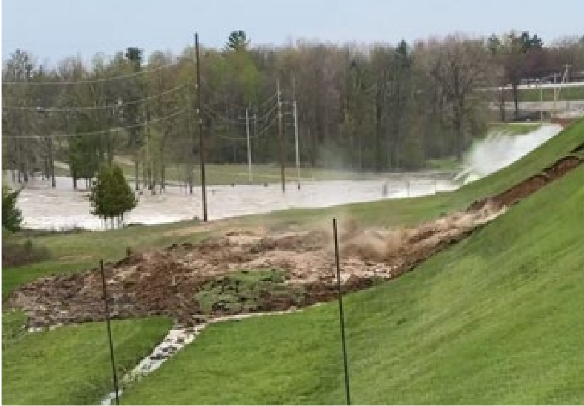
Figure 16: Enlarged still image from dam failure video at 28 seconds
