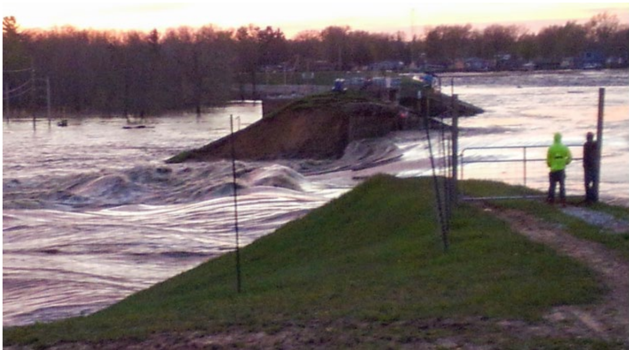
Figure 21: Edenville left embankment breach at 9:04 p.m. on Tuesday, May 19, 2020
