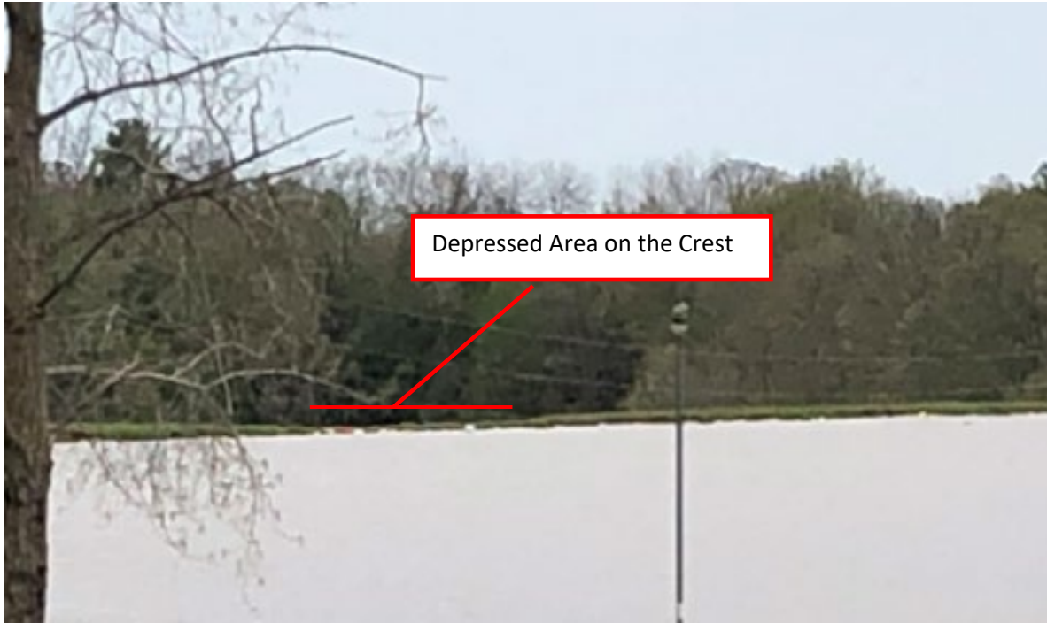
Figure 5: Photograph showing depression in the crest of the Edenville left embankment at 5:20 p.m., Tuesday, May 19, 2020
