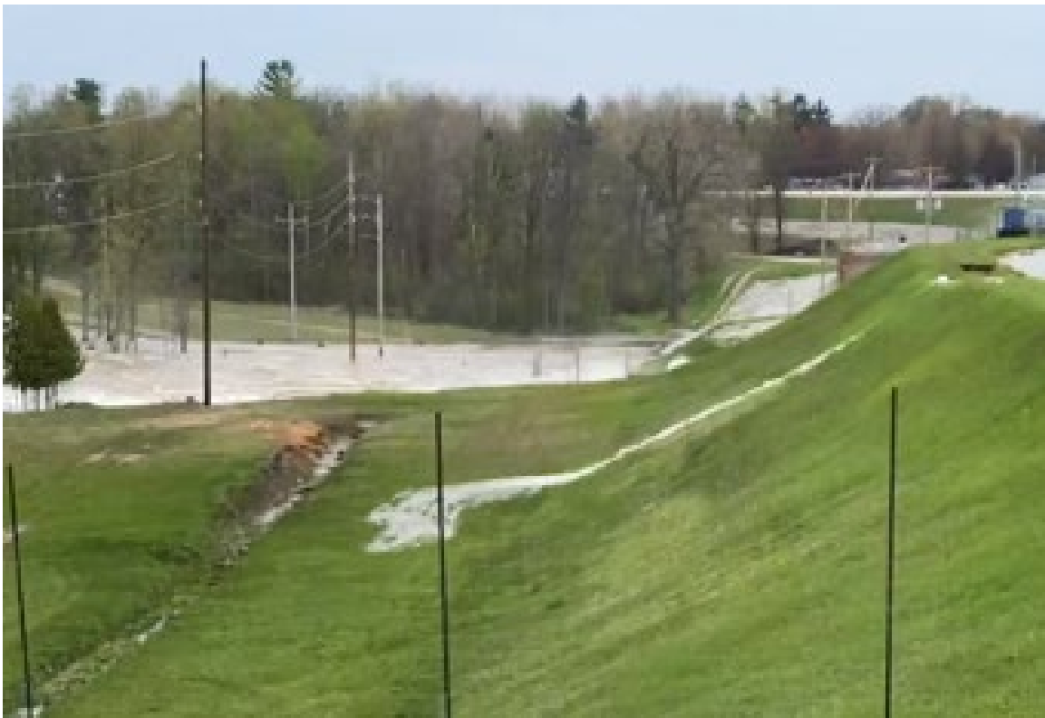
Figure 9: Enlarged still image from dam failure video at 0 seconds
