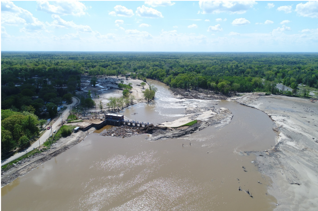
Figure 22: Sanford Dam failure, viewed from upstream (photo courtesy of EGLE)
