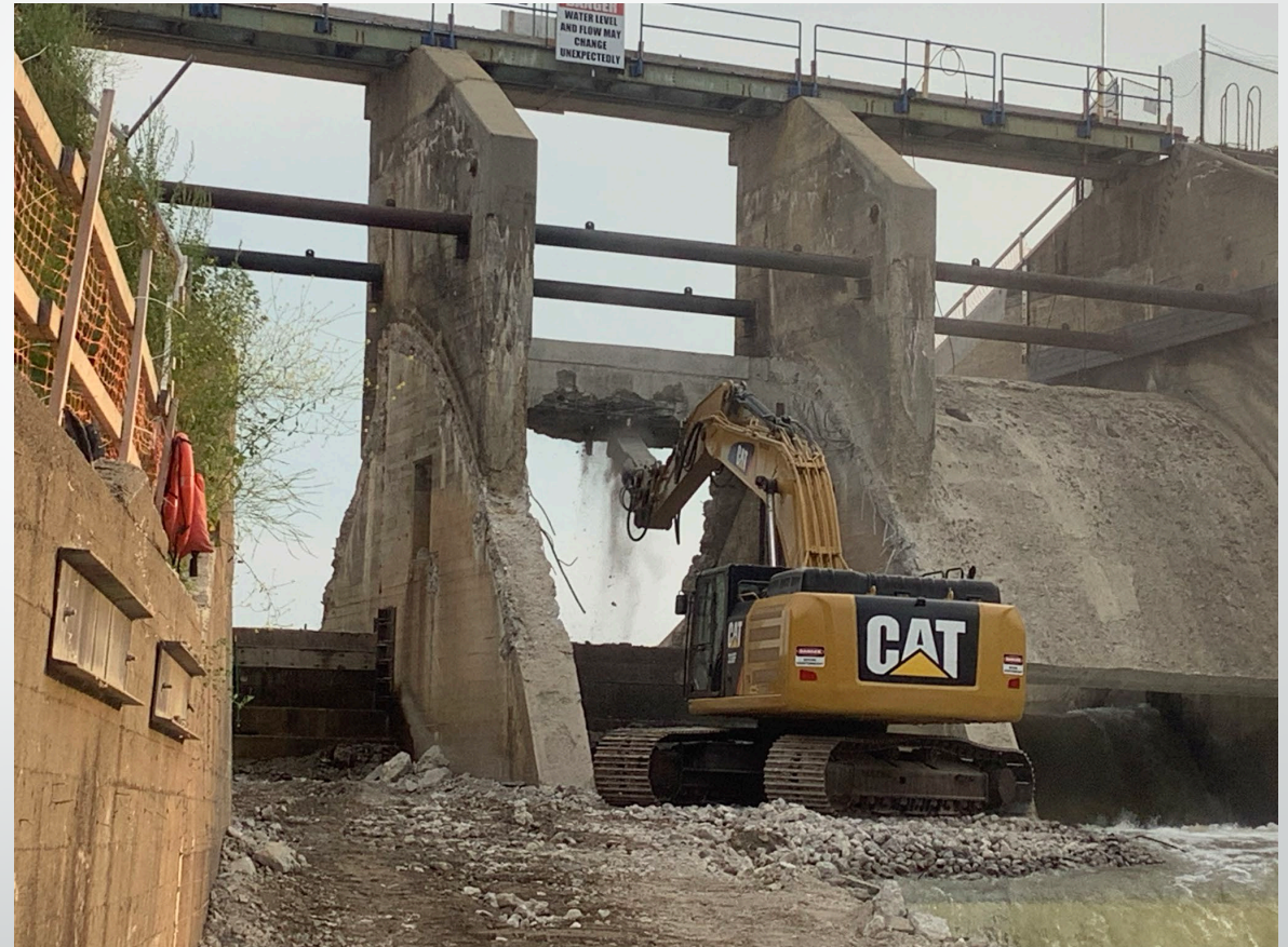
Edenville Dam, Tobacco Spillway – Spillway Demo take July 27 th , 2021
