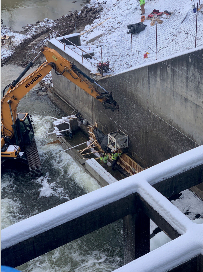
Secord Dam – Right Training wall repair
