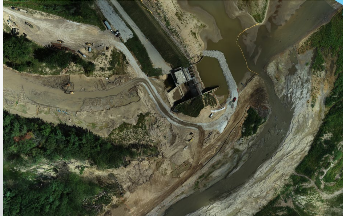
Edenville Dam – Phase II project July 30, 2021
