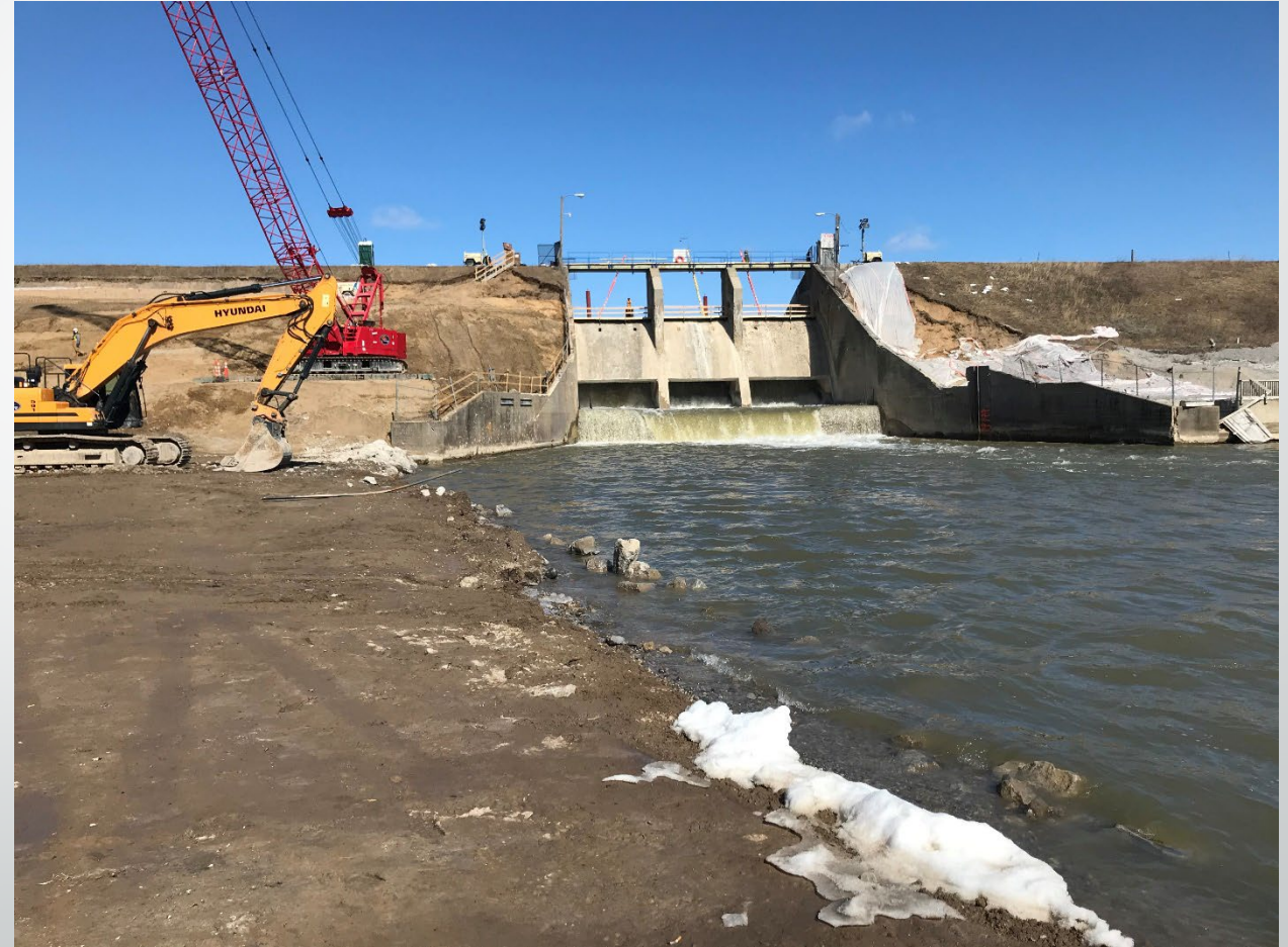
Edenville Dam, Tobacco Spillway – Looking upstream during drawdown
