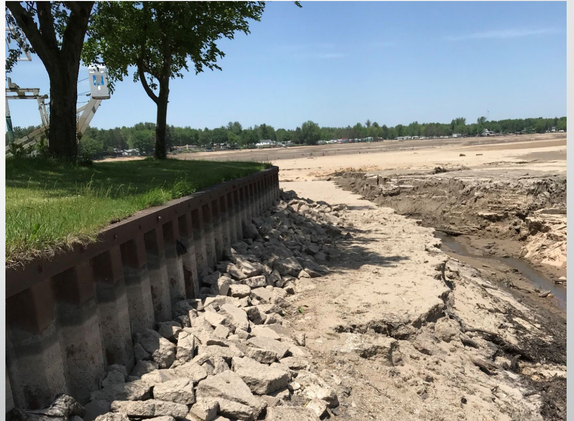
Wixom Lake –Island Drive Site, looking west. Photo taken 4/19/2020 before construction
