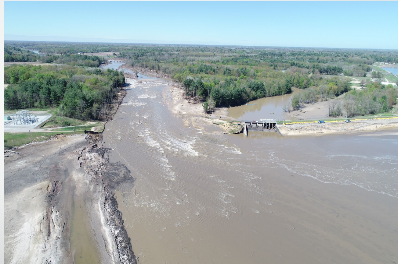
Edenville Dam – Breachway looking south. Taken May 21, 2020
