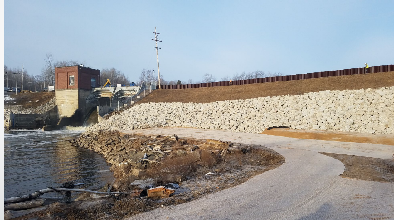
Smallwood Dam – Left embankment stabilization
