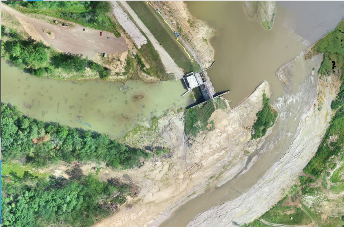
Edenville Dam – Phase II project July 14, 2021
