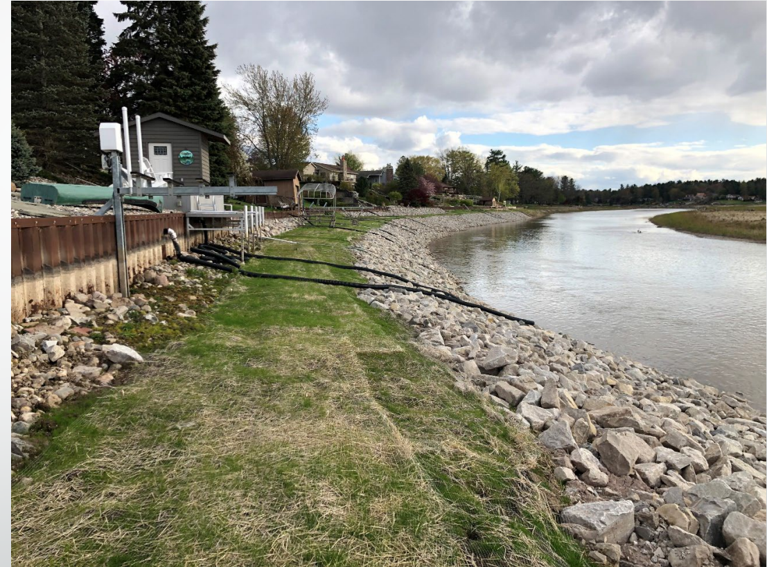
Photo taken 5/10/2021 after construction
