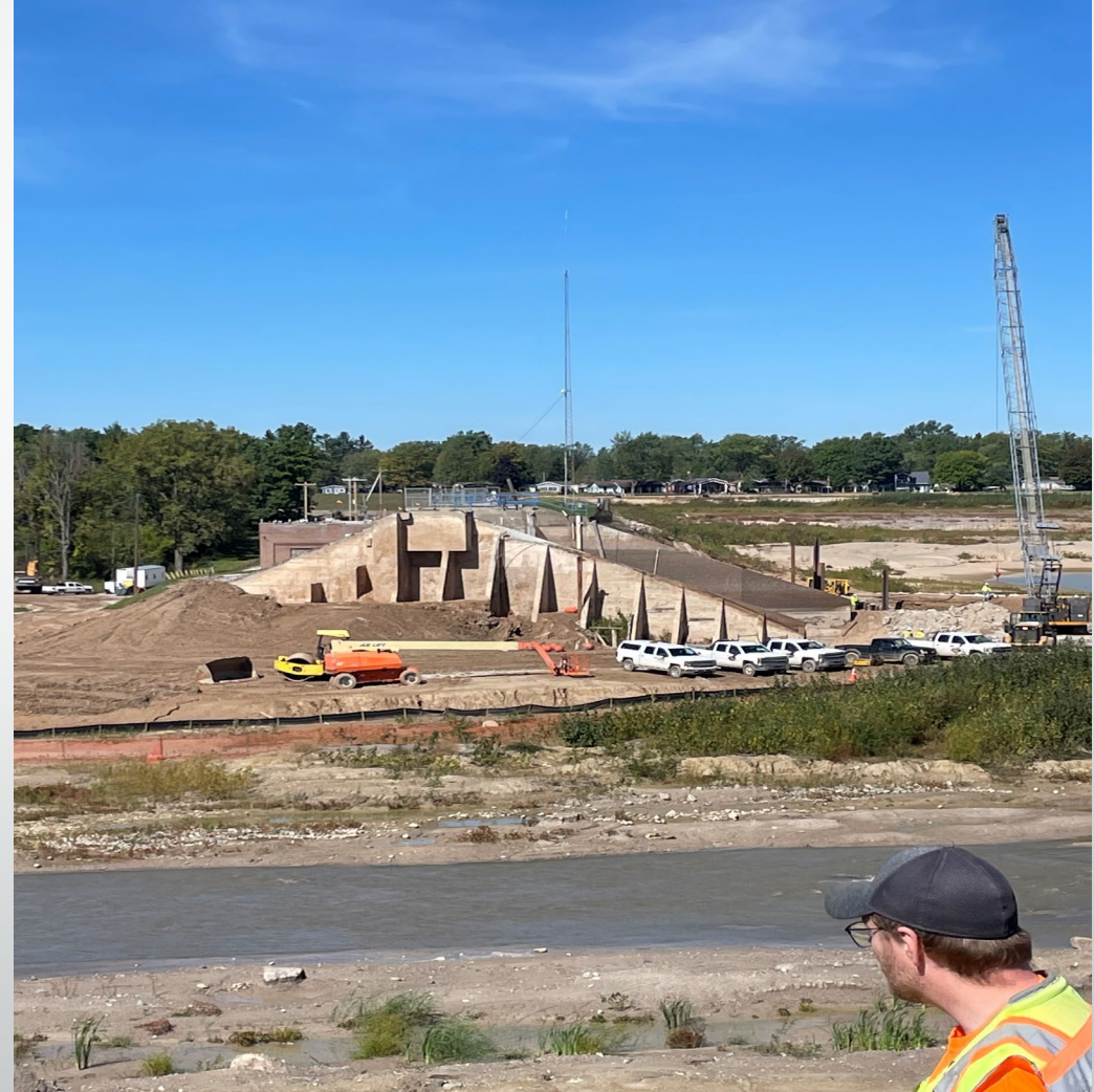
Edenville Dam – September 24, 2021. Exposed Left Side Training Wall
