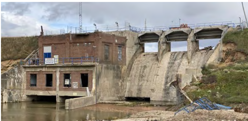
Photo 2. Tittabawasse Spillway and Powerhouse downstream, October 2020.
