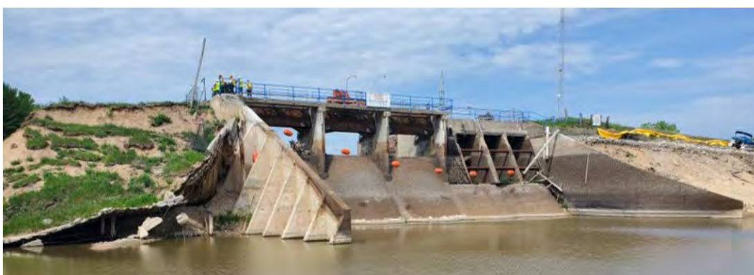
Photo 1. Tittabawasse Spillway upstream, on May 25, 2021 after completion of initial stabilization modifications.
