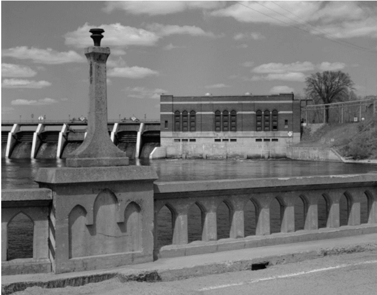
Photo 11. Chalk Hill spillway (left) and powerhouse (right).
