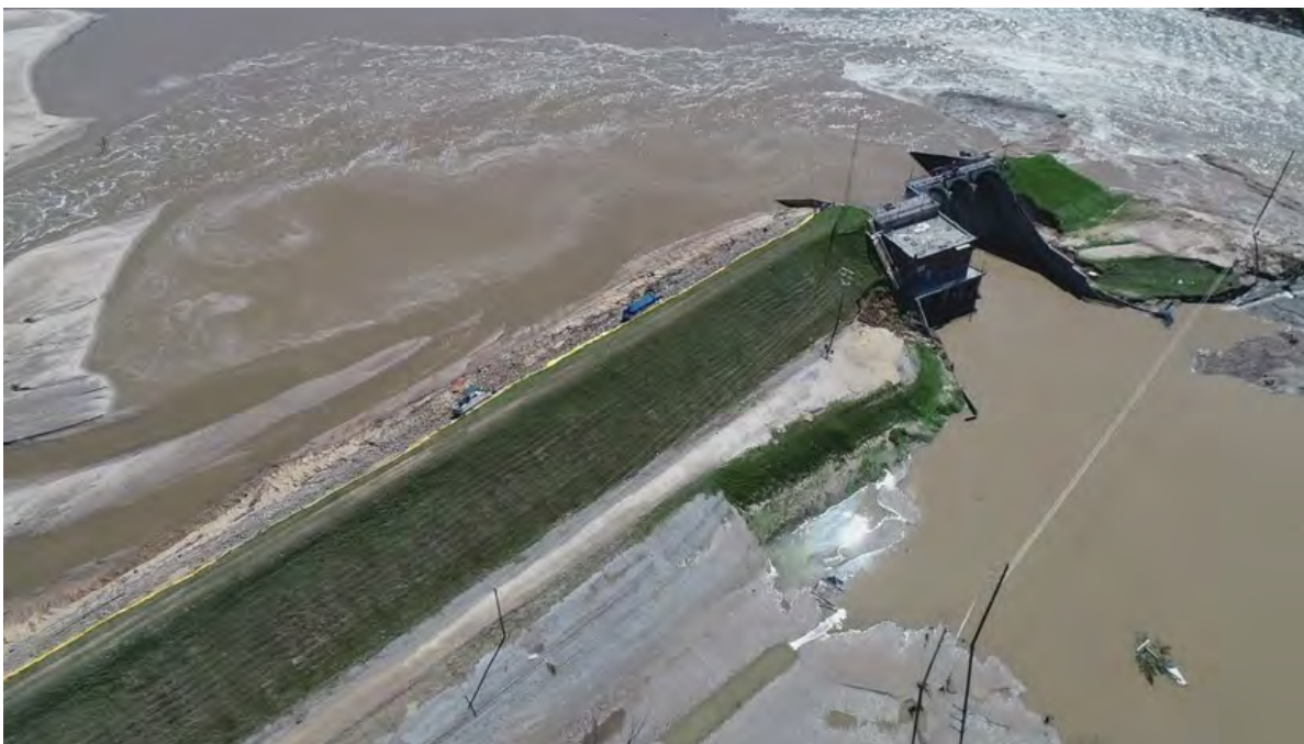
Photo 3. Left embankment along the Tittabawassee Reach of the Edenville Dam.
