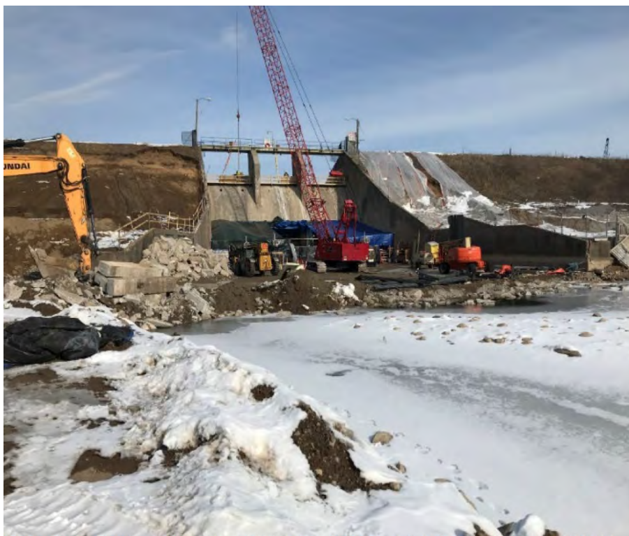
Photo 9. Phase I Interim Stabilization at Tobacco Spillway
