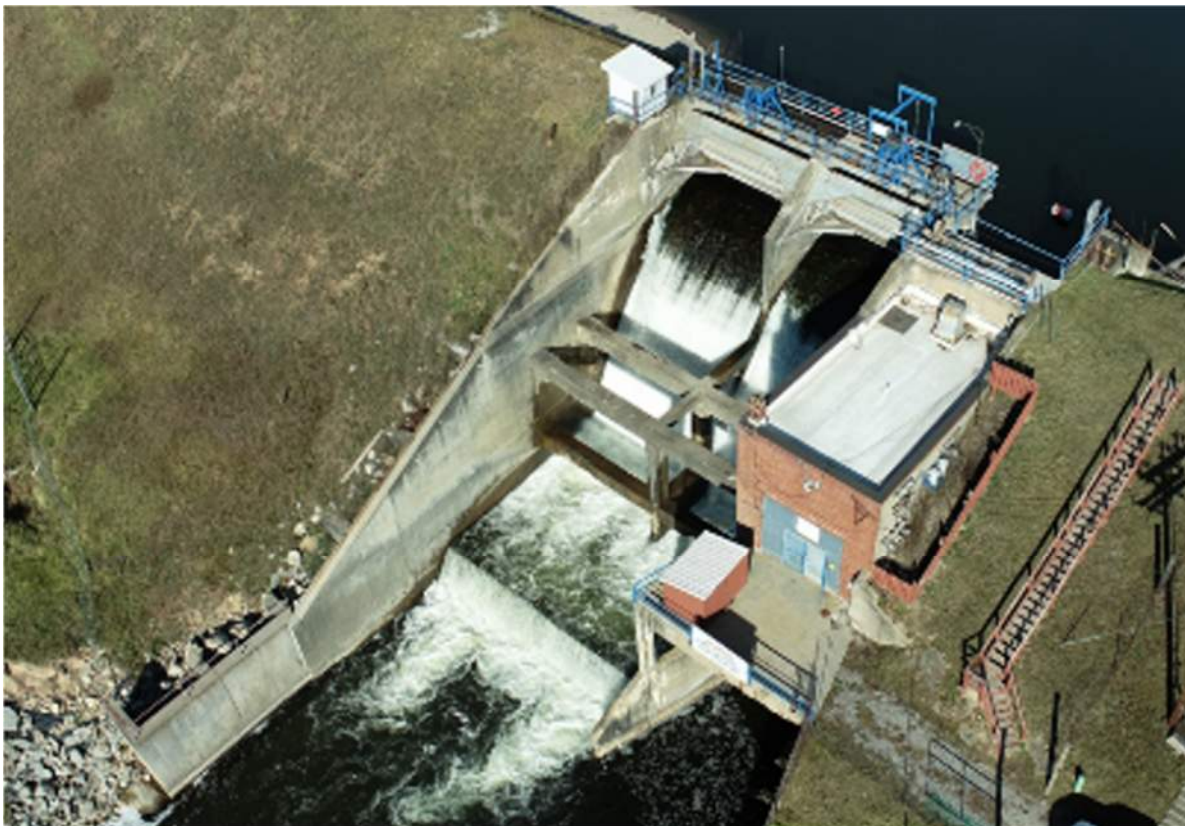
Exhibit 2 – Aerial View of Secord Dam Spillway and Non-Operational Powerhouse
