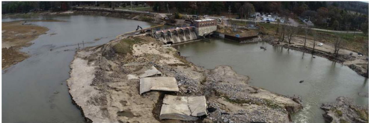
Exhibit 17 – Aerial View of Sanford Dam Failure
