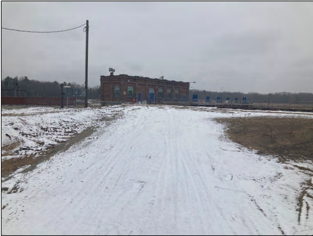
Photograph pp20 view Northwest
