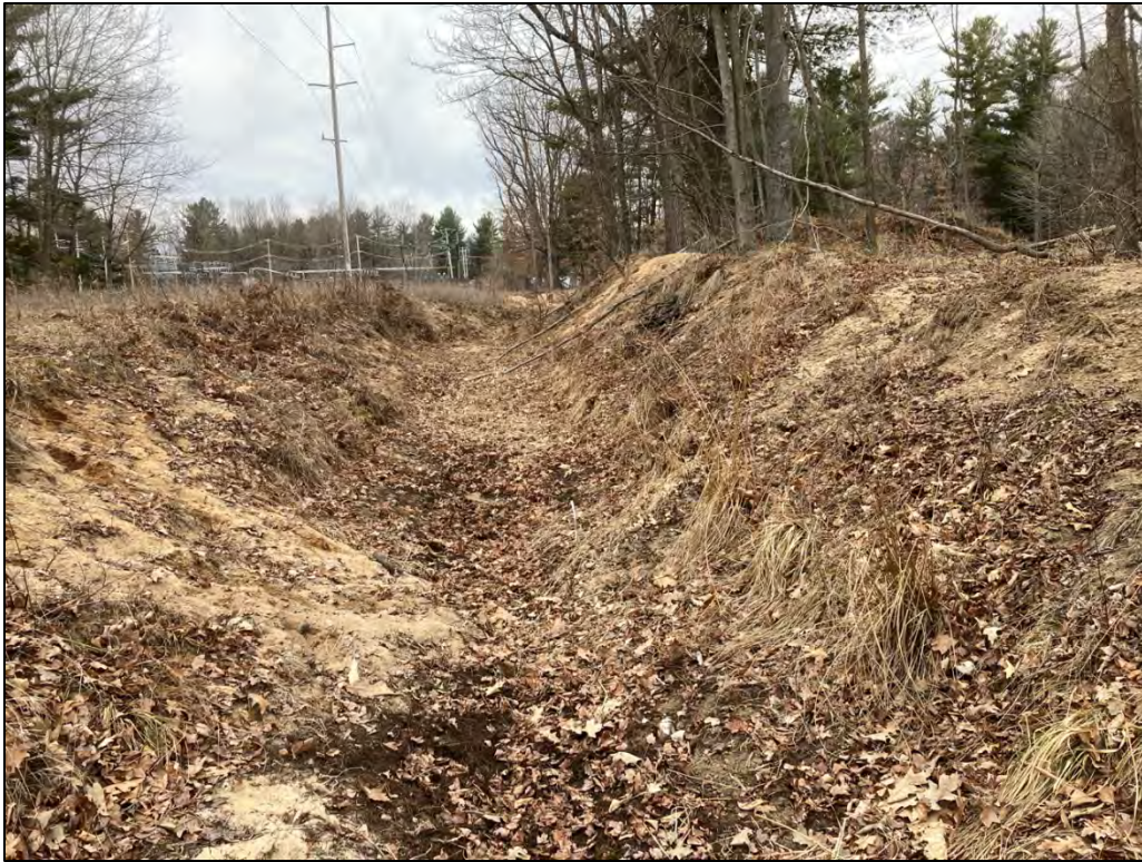
Photograph pp33 view West towards dp15
