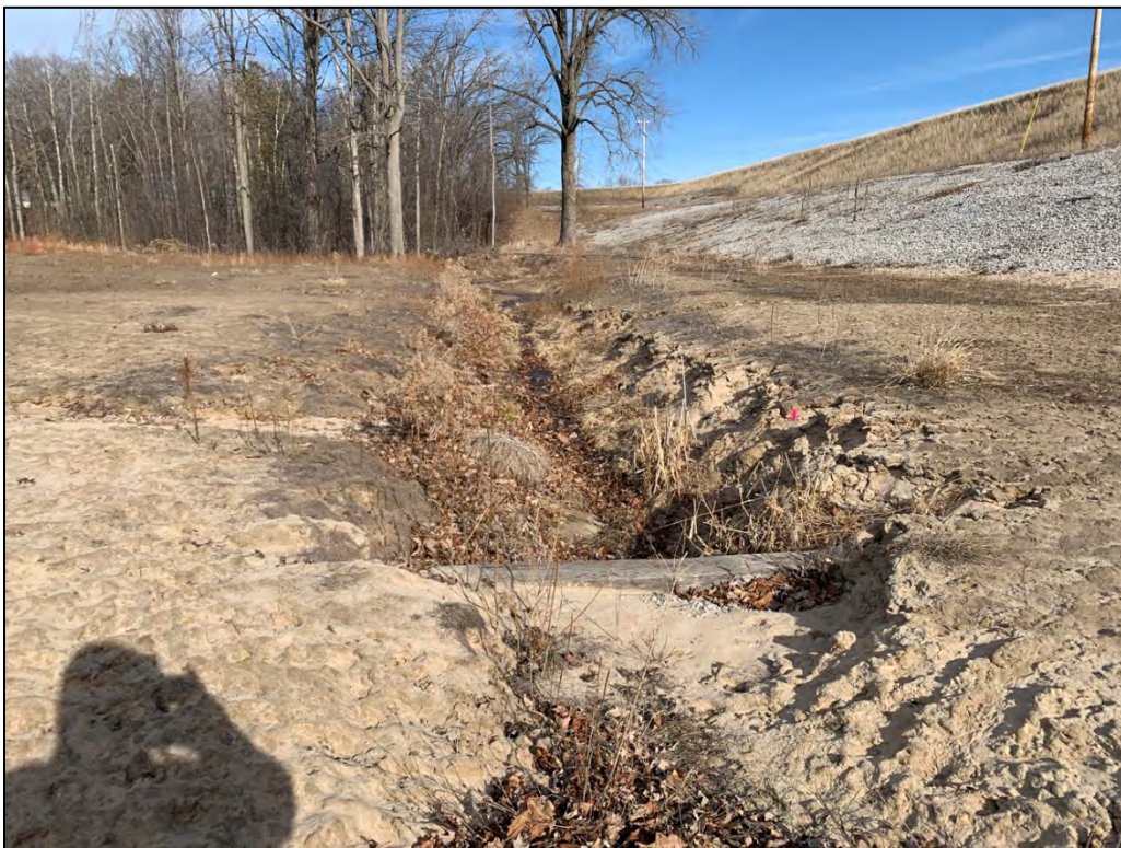
Photograph pp91 view Northwest
