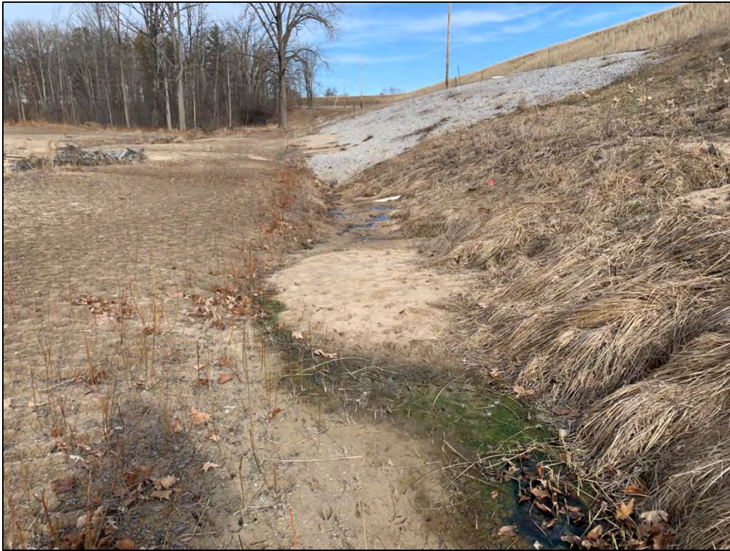
Photograph pp90 view Northwest at dp29
