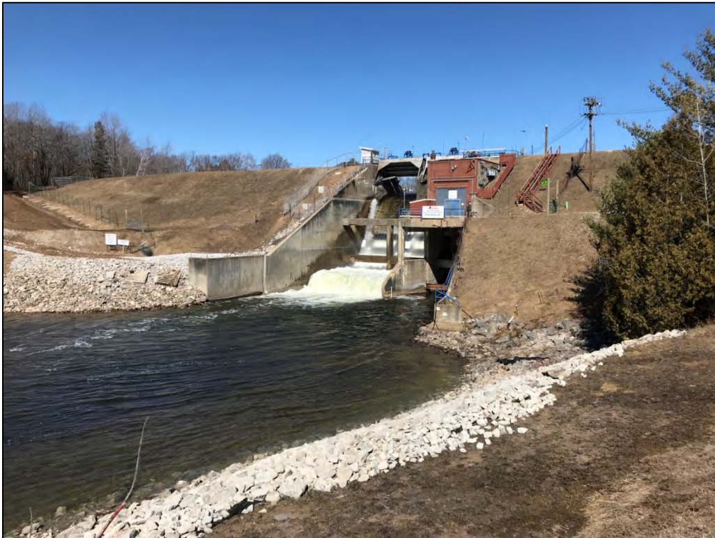
Photograph pp12 view North
