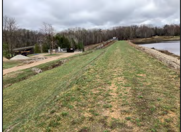
Photo 6.1-2. Eastern berm flanking Secord Dam, facing west.
