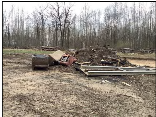
Photo 6.2-4. Clearing with refuse pile and cut tree piles, facing south.
