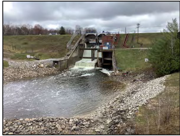
Photo 6.1-4. Secord Dam, facing north.
