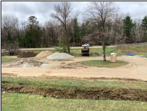
Photo 6.1-3. Secord Dam parking area, facing south.
