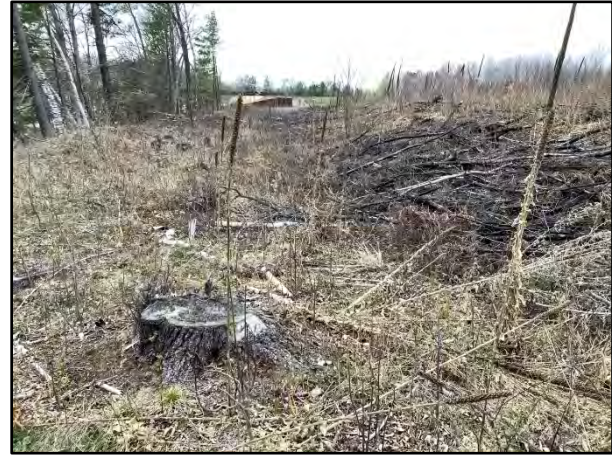
Photo 6.2-14. Woody debris from clearing, facing north.
